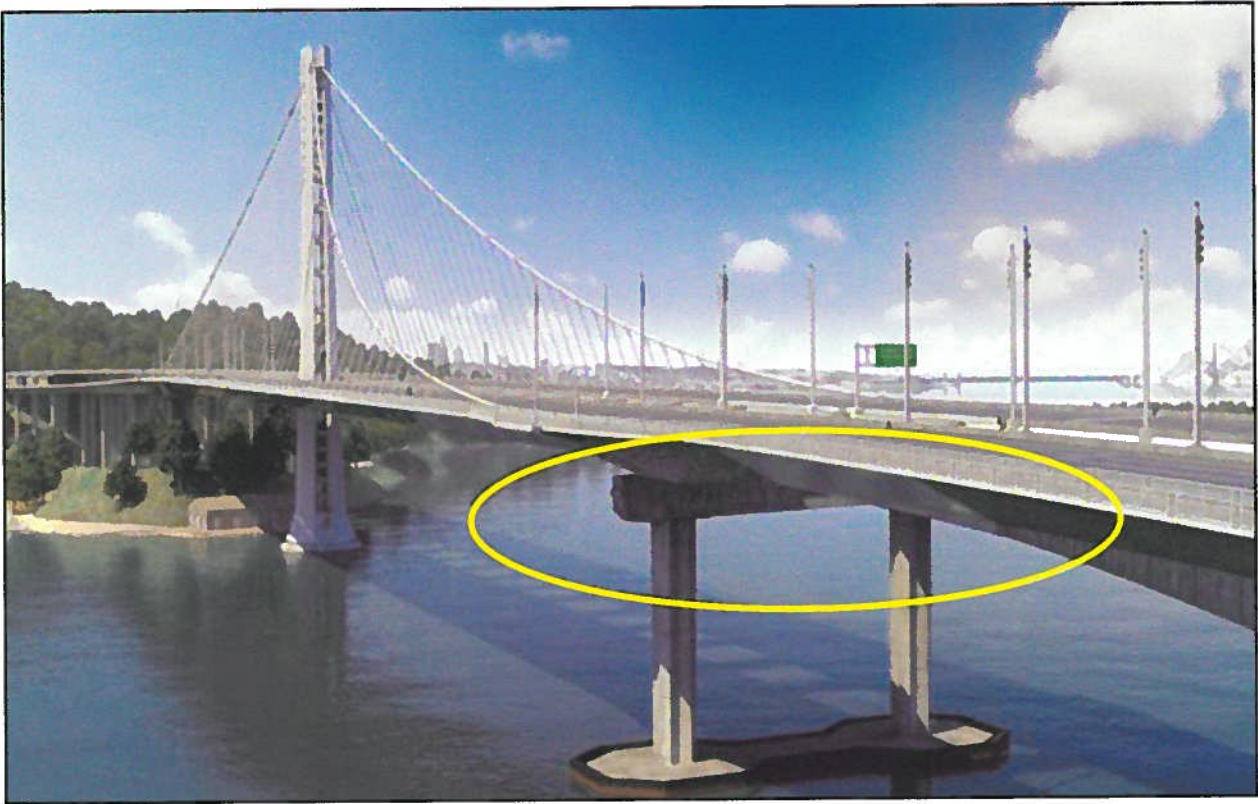
Location of Pier E2
