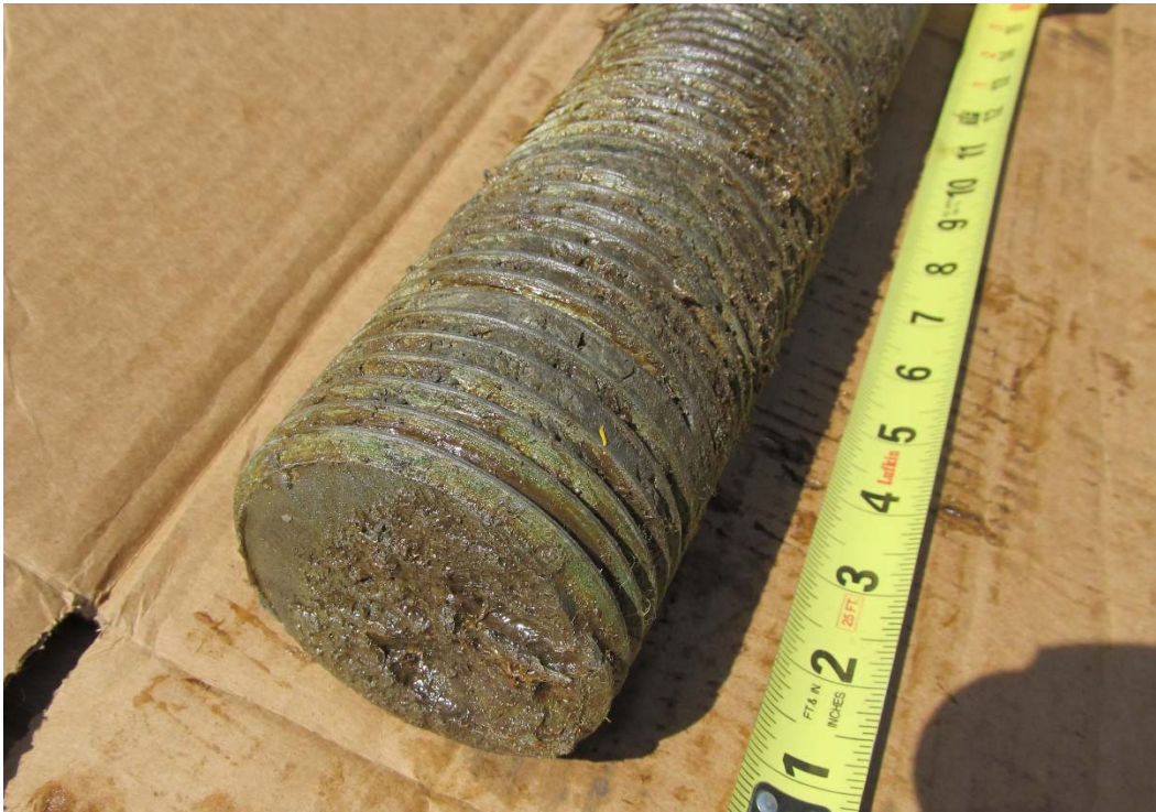
Photo 2) Broken anchor rod S1-G1.
