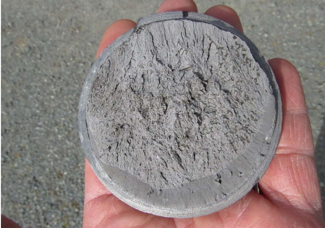
Photo 7) Fracture surface of Rod S2-A6 after cleaning.
