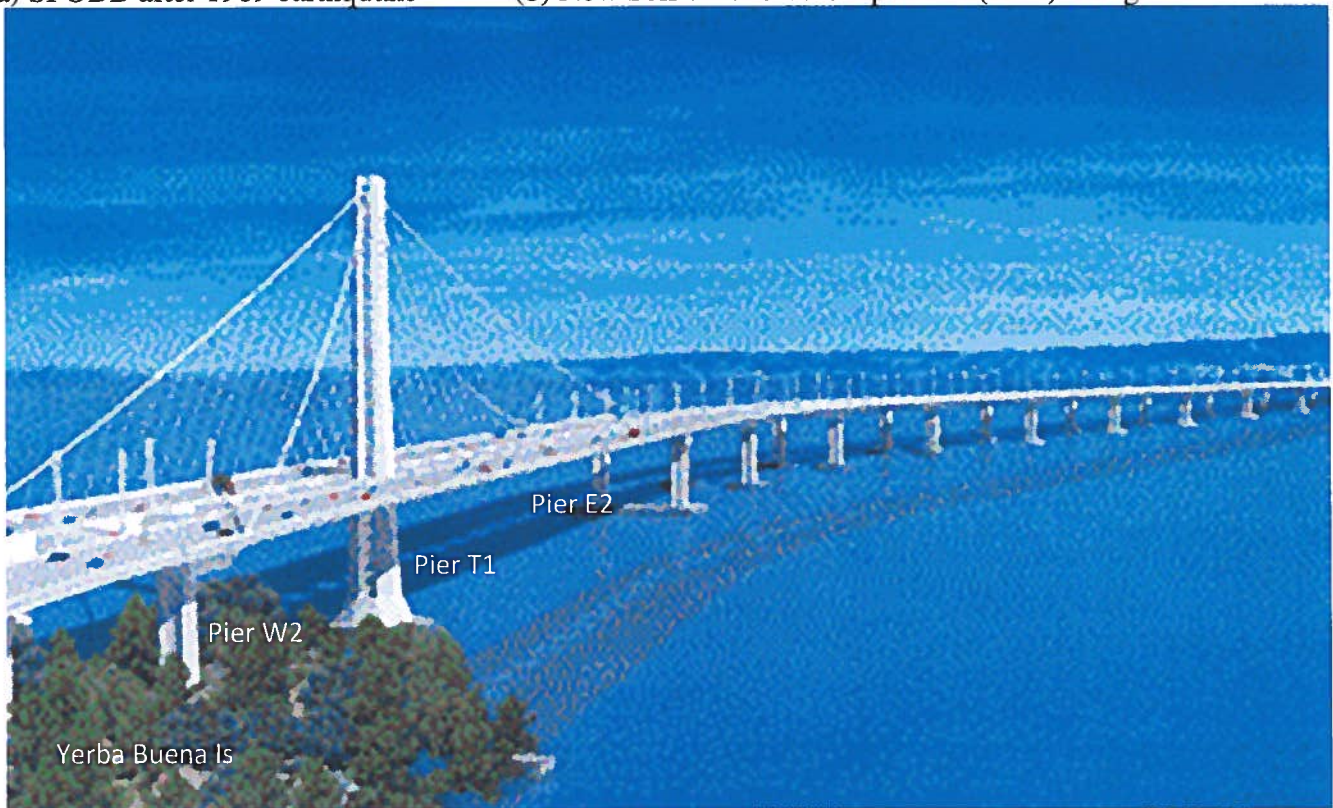
(c) Piers T1, E2, and W2 of SAS Bridge
