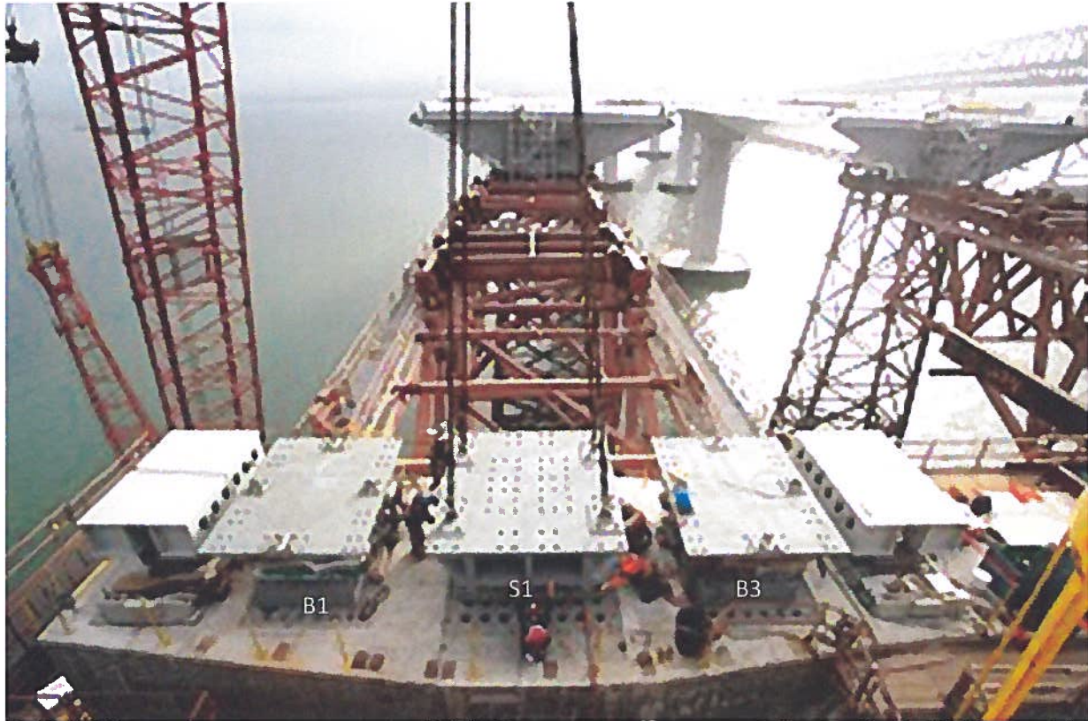
(a) Top of Pier E2 Cap Beam after installing B1, S1, and B3
