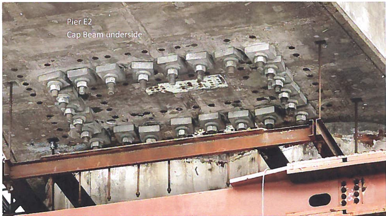
(b) Underside of the Pier E2 camp beam showing anchor rods for a bearing
