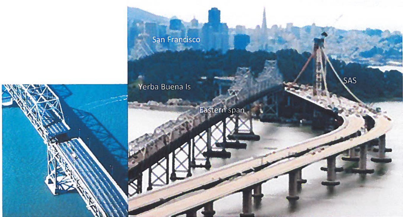
(a) SFOBB after 1989 earthquake
