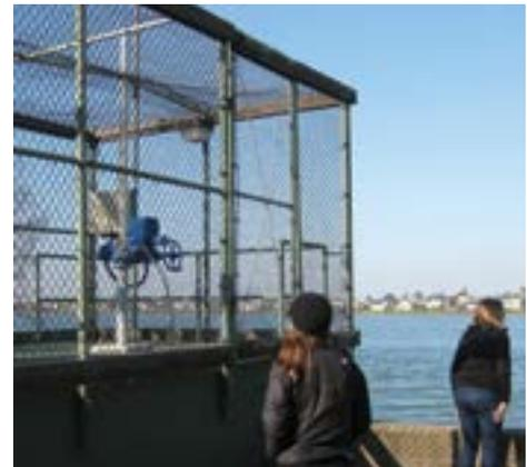
*Bay Farm Isle pump station, one of hundreds of aging facilities around the region used to keep our communities and shorelines dry. Many are under-sized, at capacity, and at the end of their service lives. To cope with SLR and storms, they need upgrades, maintenance, and back up power. Photo from archives.*
