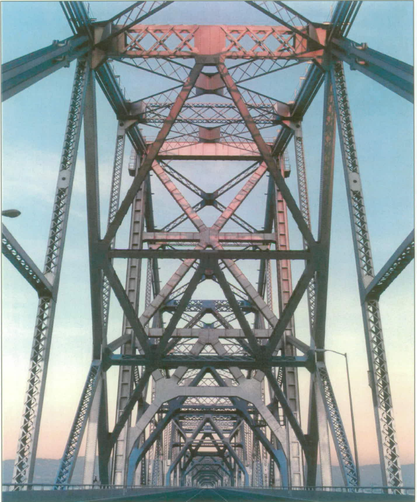
East span superstructure from within the cantilever section looking east. Note the number of pieces. Each connection and member is an opportunity for failure. Some members have multiple failure mechanisms.
