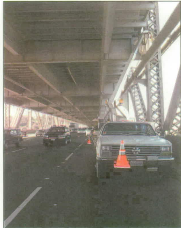
Truss construction modifications adjacent to traffic
