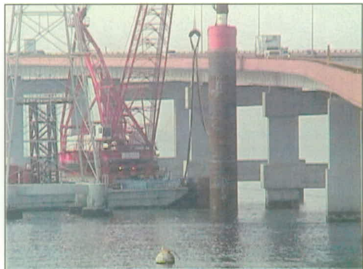
Pile installation at San Mateo-Hayward Bridge
