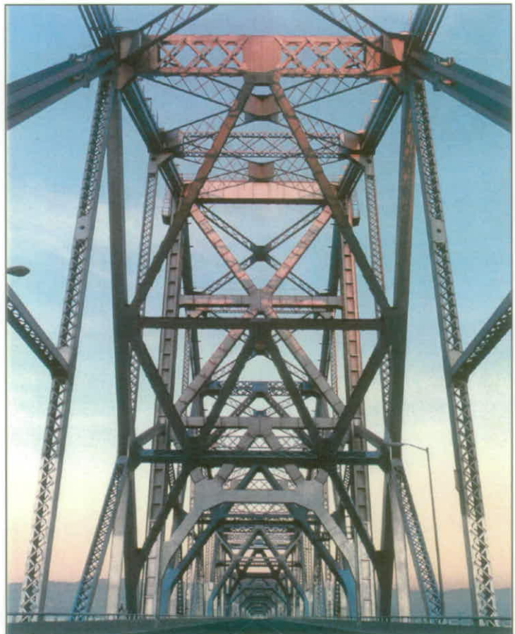
Cantilever truss member and elements on the East Span
