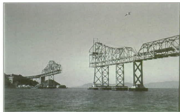
Construction of the Cantilever Section
