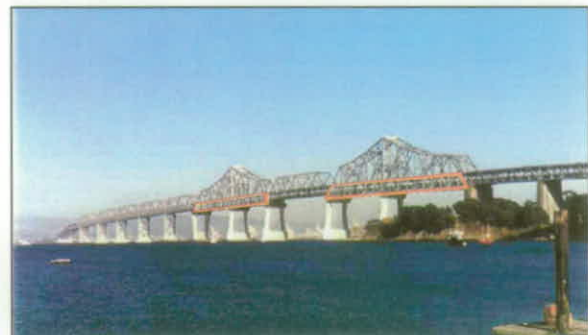
Cantilever with two new support towers (external steel truss outlined in orange)
