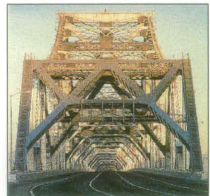
Cantilever section on the east span
