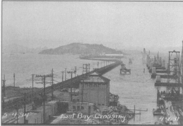
Foundation construction near the Key System pier
