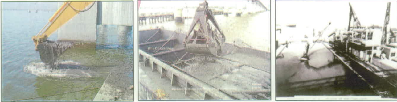
Dredging techniques – backhoe, clamshell, hydraulic
