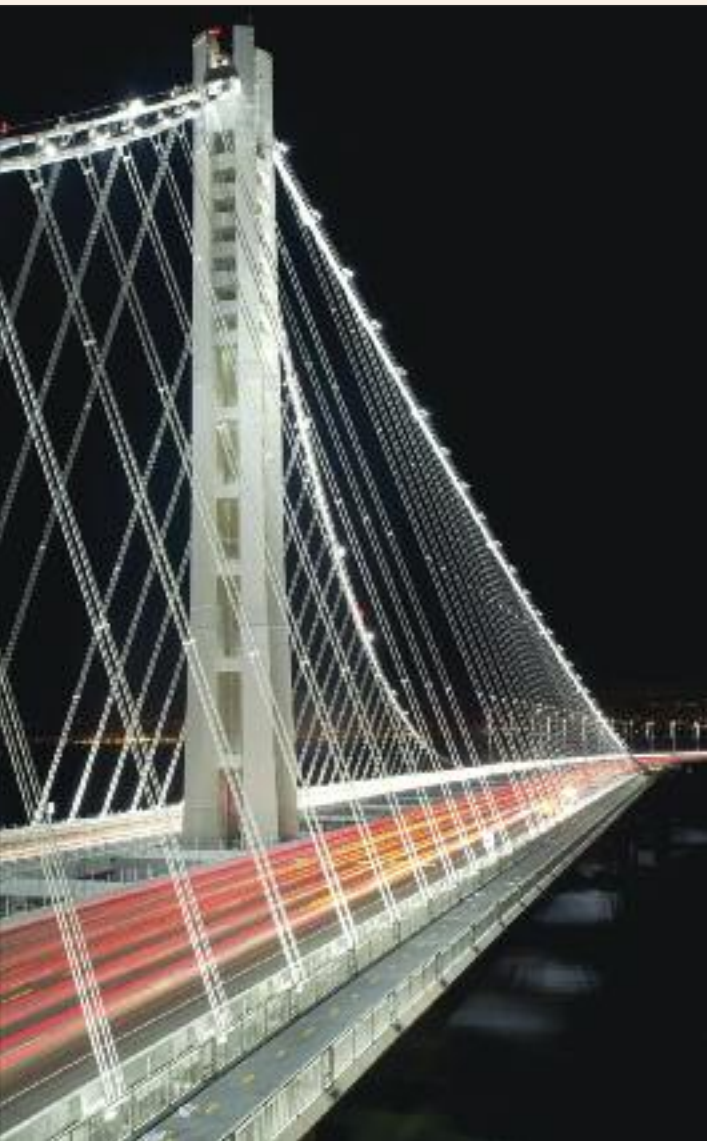
The New East Span of the San Francisco-Oakland Bay Bridge opened on Labor Day 2013. (Photo: Noah Berger)
