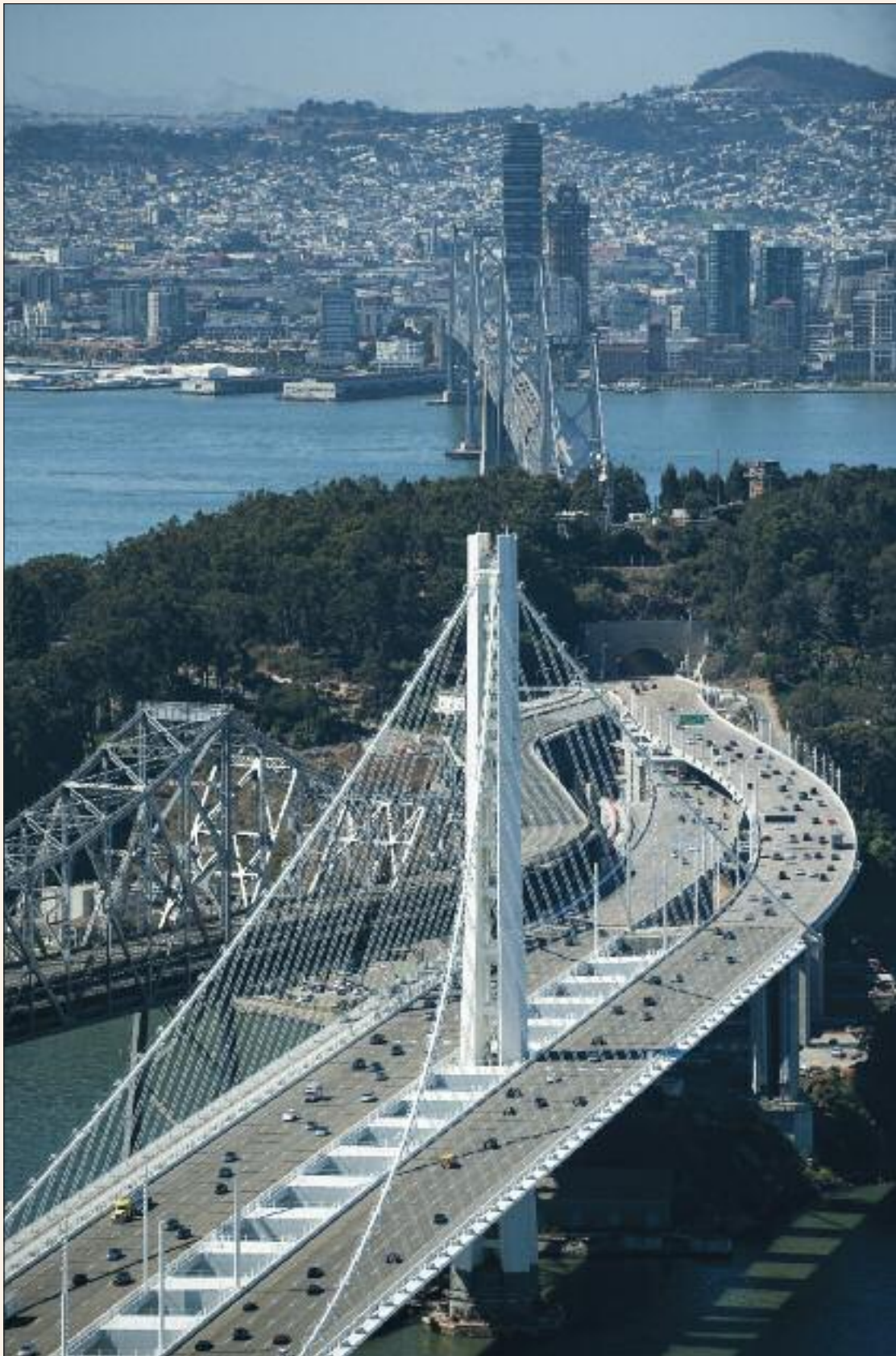
The TBSRP included both the new Bay Bridge East Span and a retrofit of the West Span. (Photo: ©Barrie Rokeach 2014, www.rokeachphoto.com )
