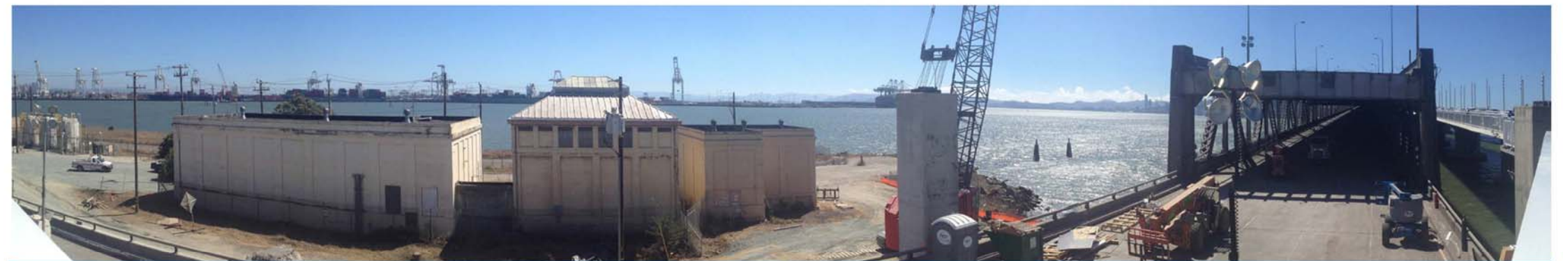
Looking south at the historical buildings at the mole from the elevated bike/ped path
