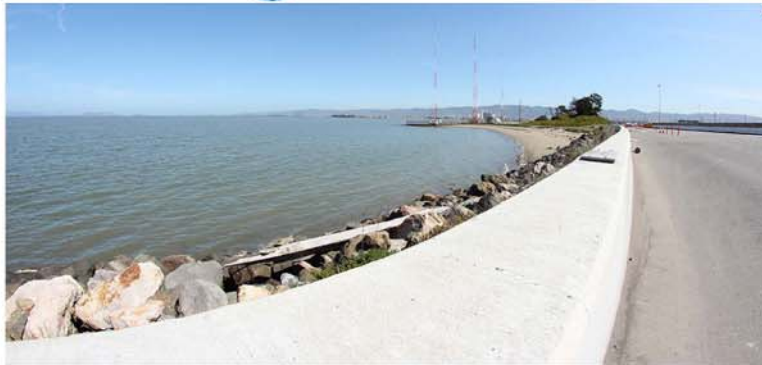
Looking east at Little Radio Beach
