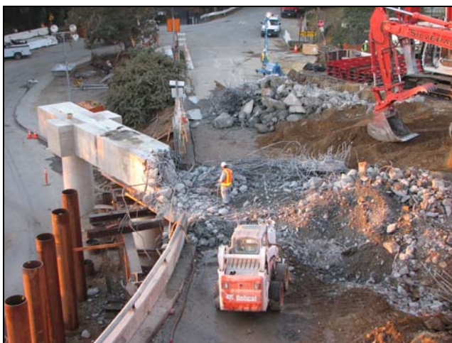
Demo of the Skid Beam on the Ramp 9/3/07 Early Morning
