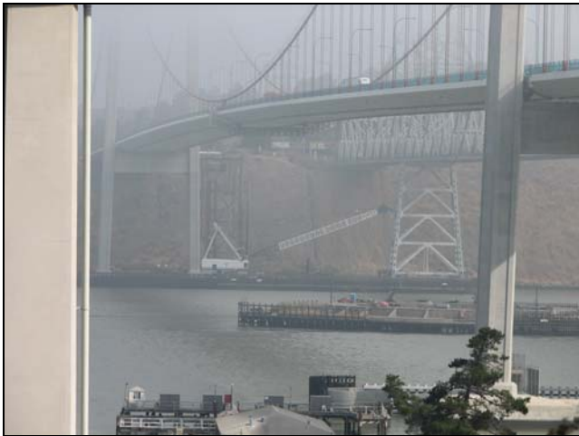
Looking North at the Demolished Carquinez Bridge
