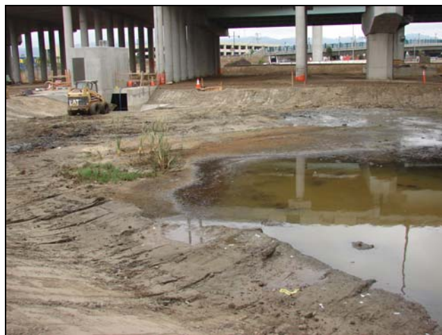
Area 5 – Forebay Detention Basin
