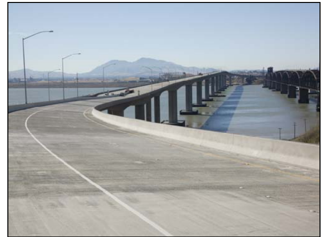
The New Deck Looking South
