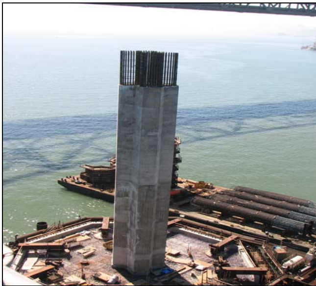
E2-T1 - Eastbound Column at E2
