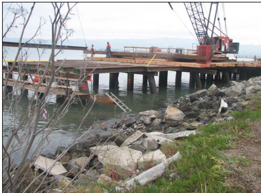
OTD #1 Trestle Construction
