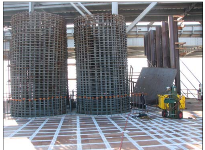
SAS - Top of W2R Column Reinforcement
