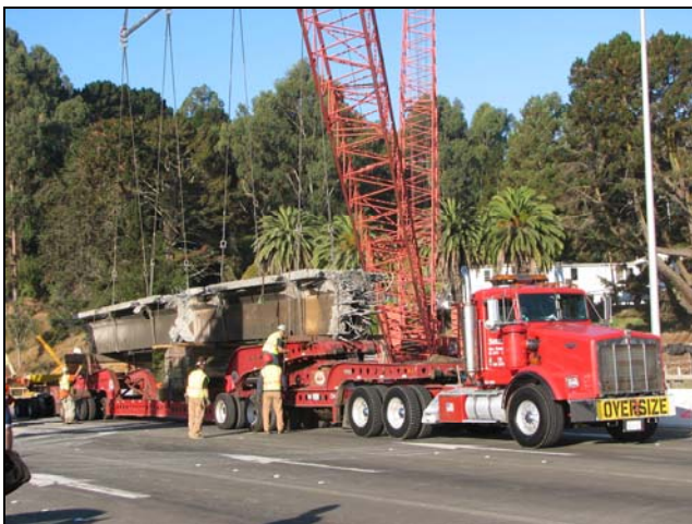
Loading Demolished Girder on the Truck 3pm 9/1/07
