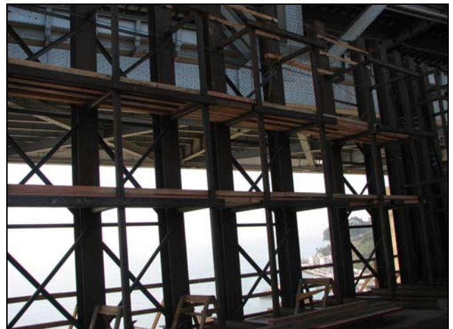
SAS - W2 Bent Cap Forms
