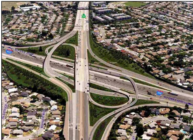
Interstate 880/State Route 92 Interchange AFTER
