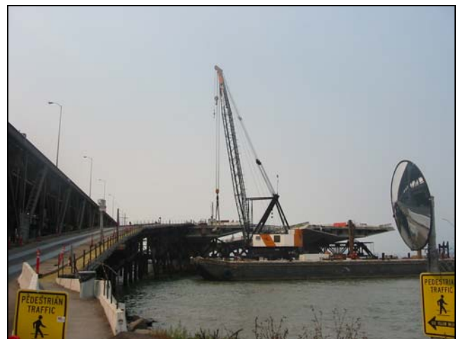
Skyway - Installing Hinge Pipe Beam E - Eastbound (1)
