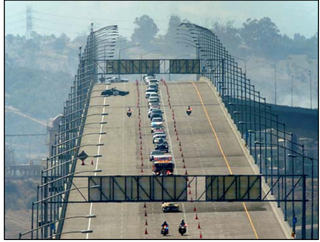
The First Convoy of Cars Inaugurates the New Span
