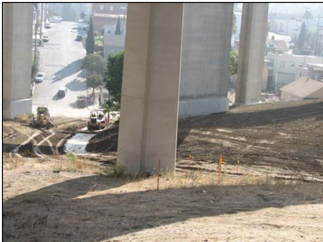
The East End of the Wanda Street Realignment
