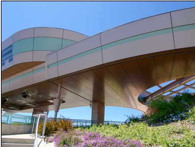
The New Toll Plaza
