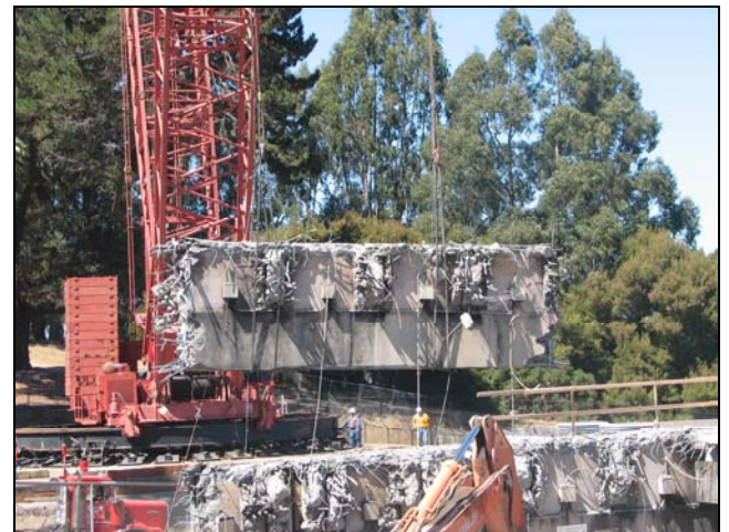
Lifting a North Edge Girder 5:30pm 9/2/07
