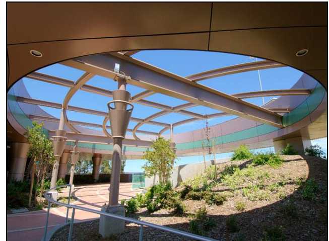
Under the New Toll Plaza
