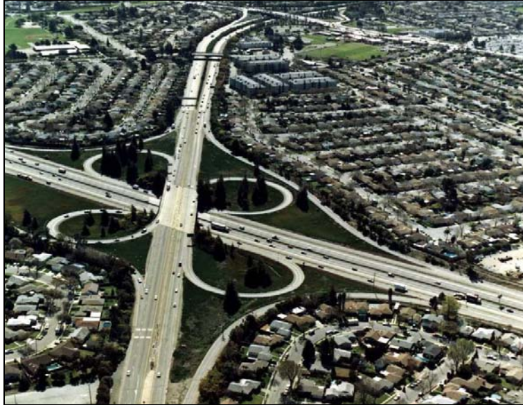
Interstate 880/State Route 92 Interchange BEFORE
