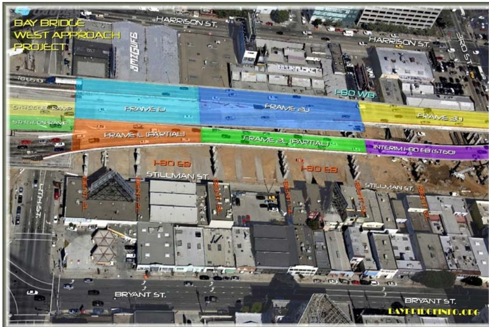
West Approach Interim I-80 Eastbound
