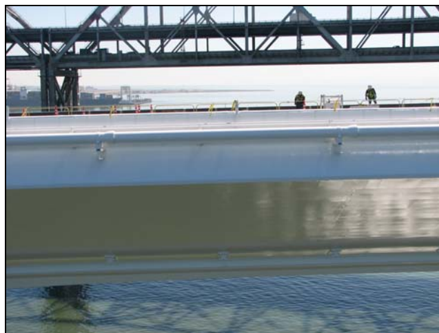
Skyway - White Painted OBG - Eastbound
