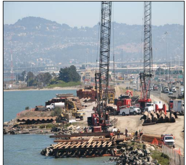
OTD1 - Construction of the Trestle
