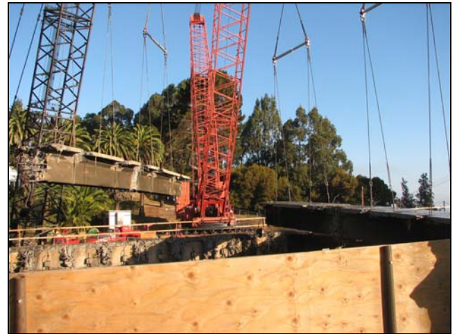
Lifting of Two Girders 2pm 9/1/07
