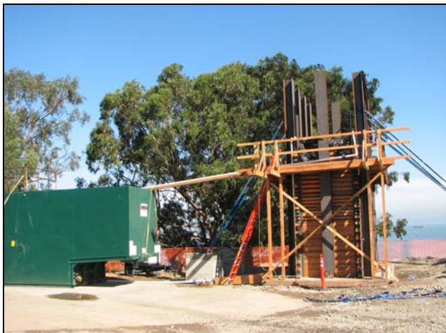
SAS - Mass Concrete Mock-up with Cooling System
