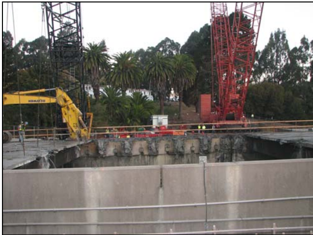
Seven Girders Removed 11am 9/01/07
