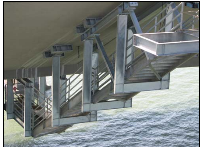
Skyway - Stairs Leading to the Substation
