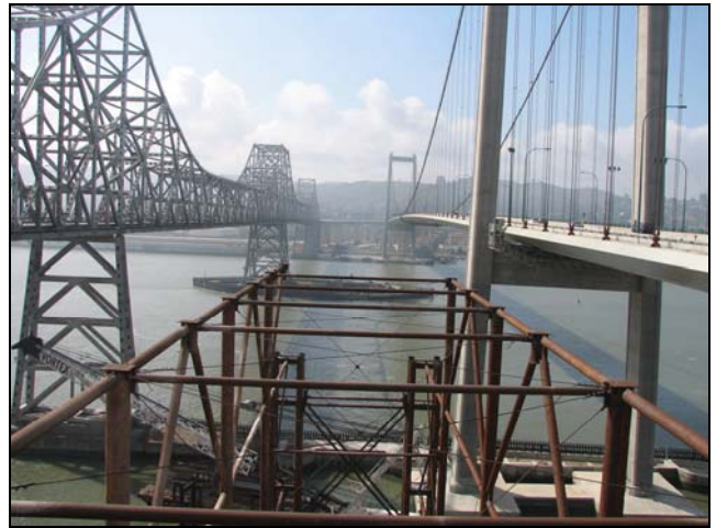
Looking South of the Recently Demolished 1927 Carquinez Bridge
