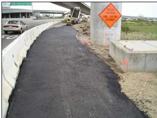
A7 Line - AC Paving
