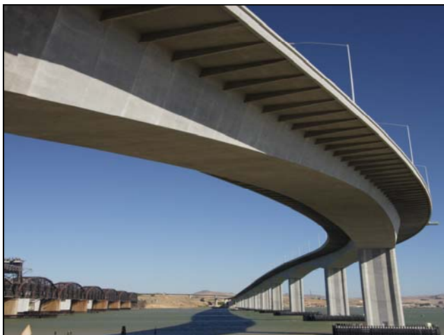
The New Bridge Looking North
