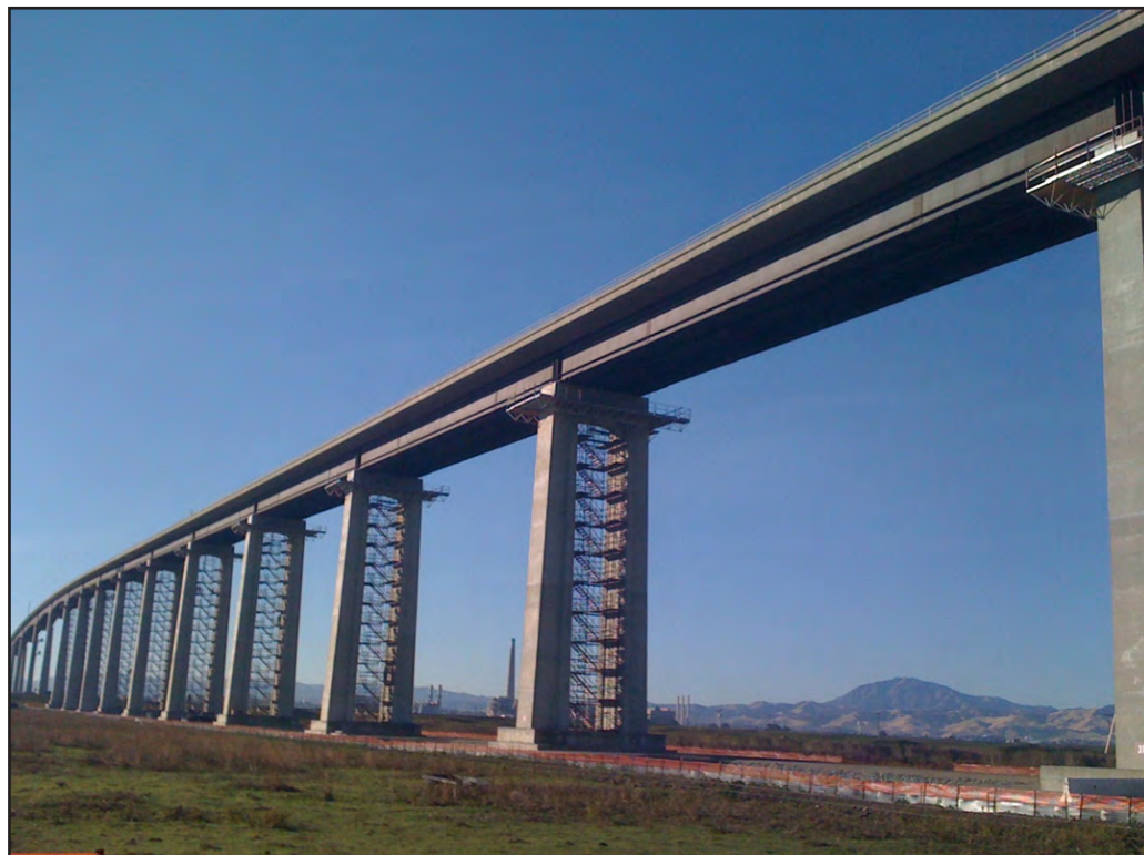
Piers Being Fitted for Construction Access Scaffolding
