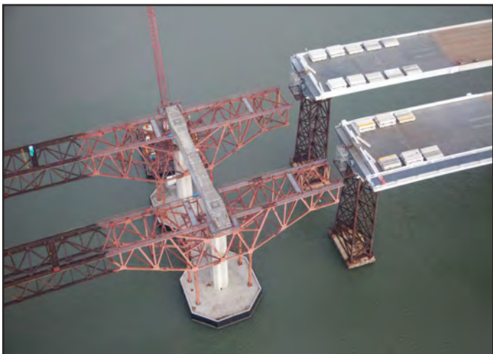
SAS E2 Cap Beam and the end of the Skyway
