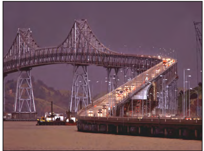
Richmond-San Rafael Bridge
