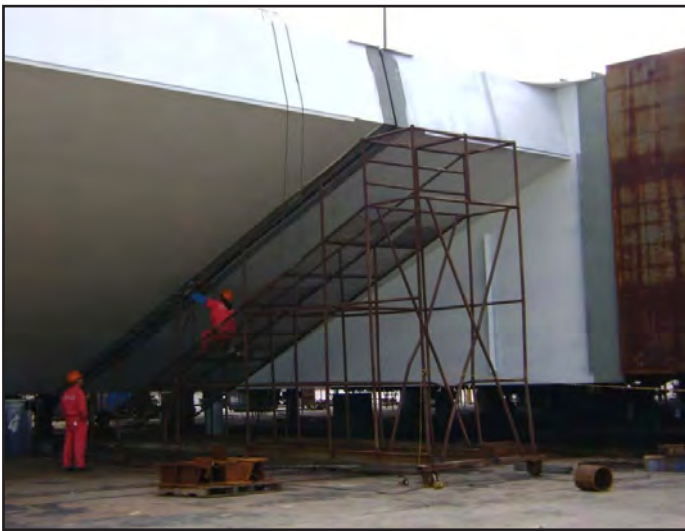
SAS Roadway Box Segments - Lift 11 in Trial Assembly Yard
