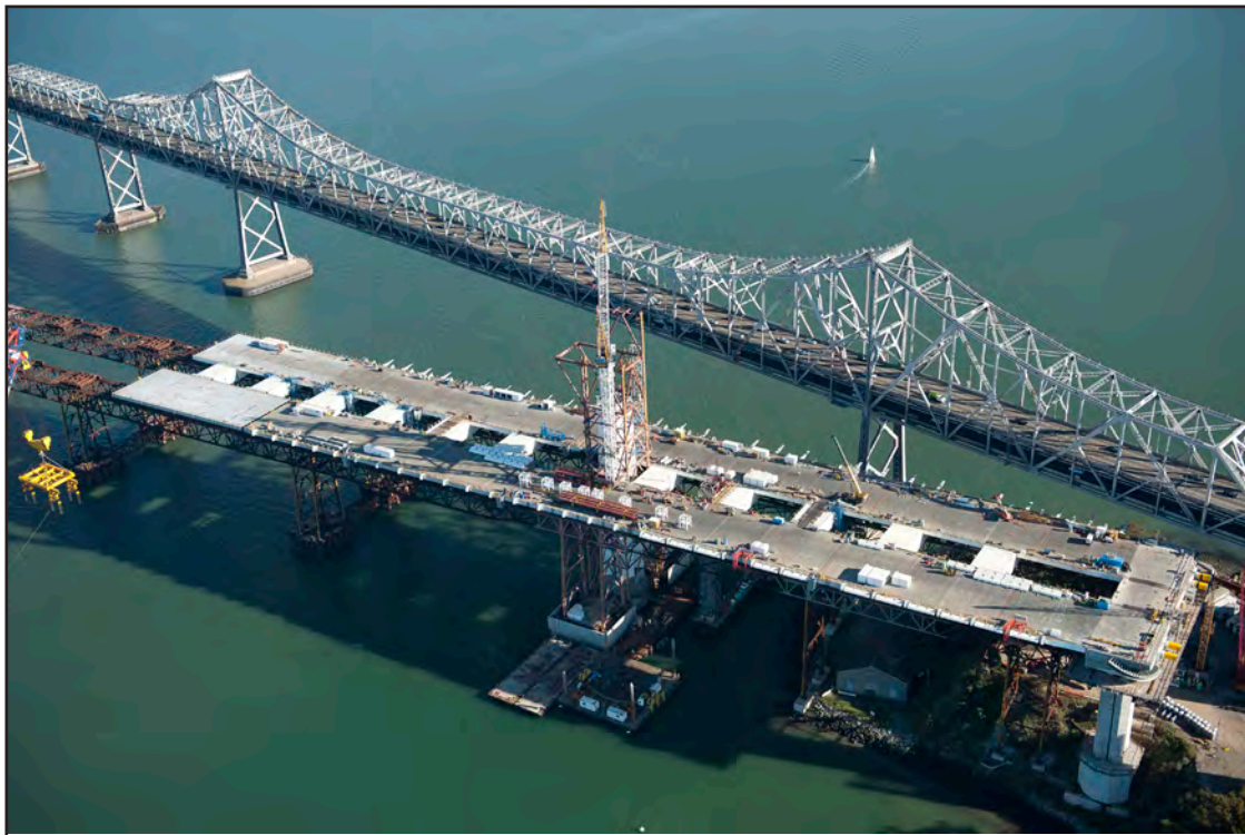
Overview of Progress of Roadway Boxes Eastbound and Westbound
