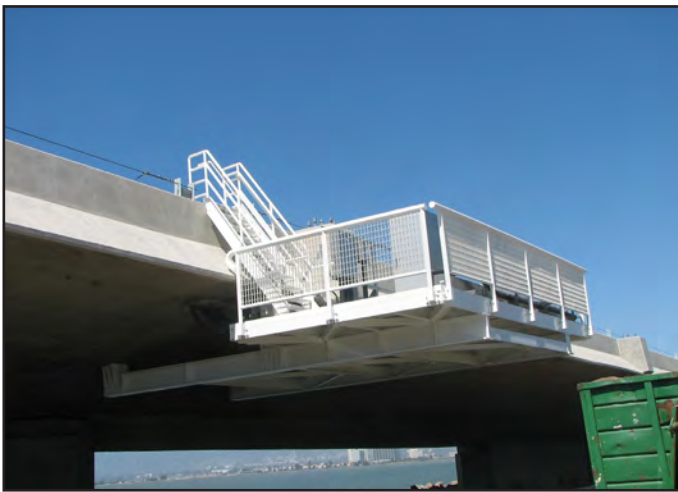
Oakland Touchdown Service Platforms Installed
