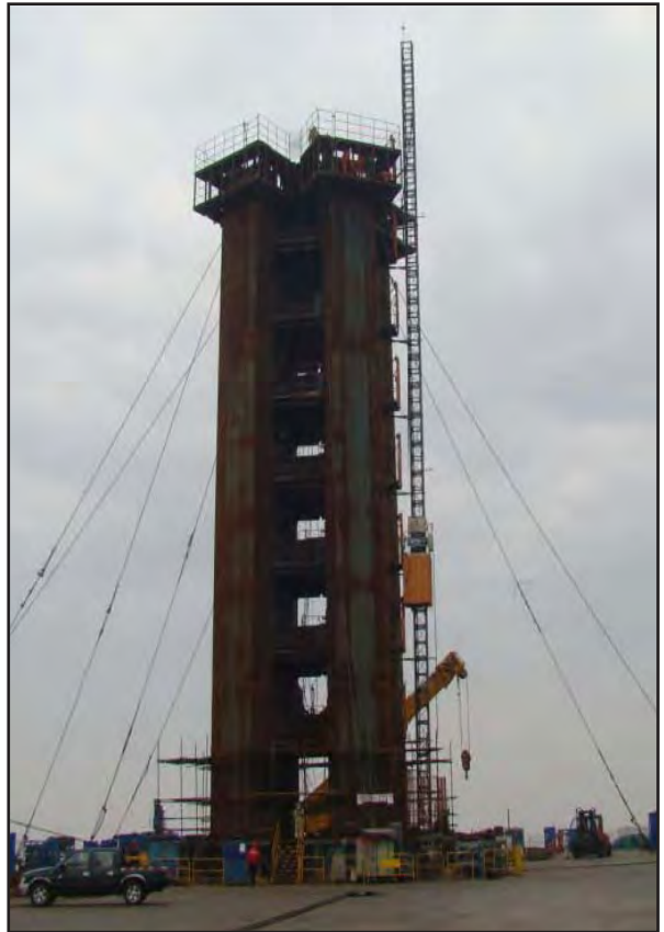
SAS Tower Lift 4 Shafts in Trial Assembly with Grillage
