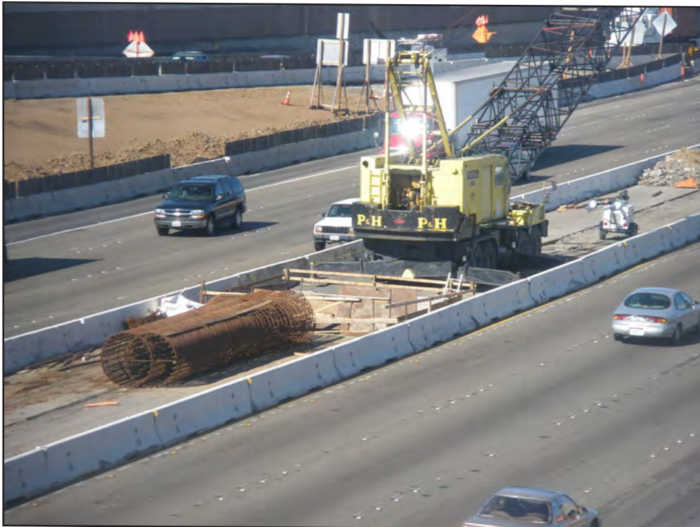
Bent 3 of WSCONN Bridge
