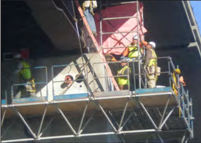
Antioch Bridge Position of Vertical Stiffeners
