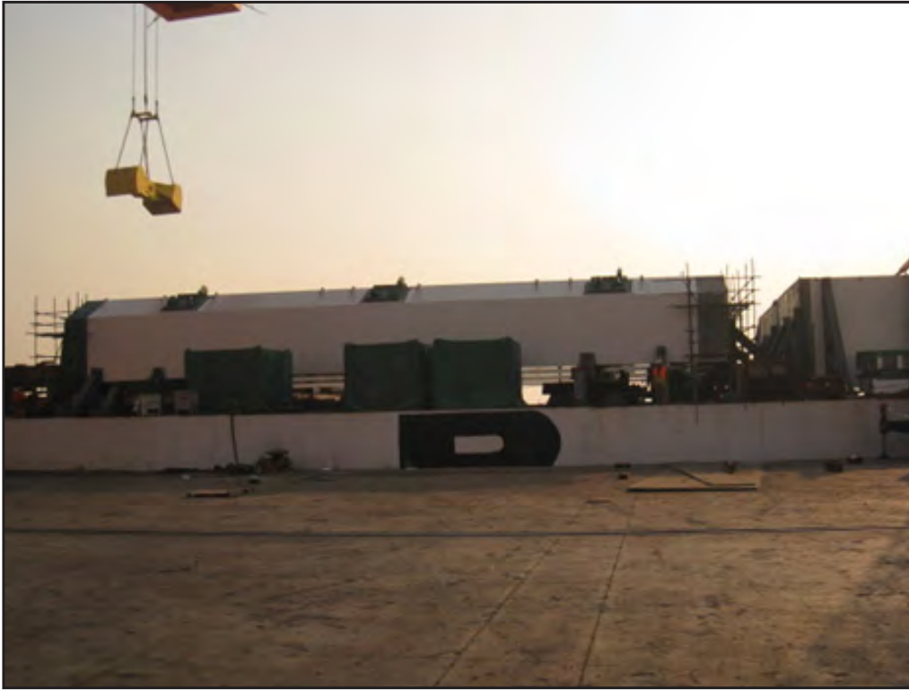
SAS Tower Lift 3 Segments Loaded up on the Ship
