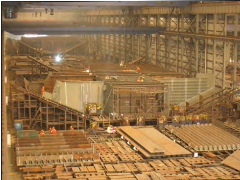
SAS Lift 13 West Line Segment Assembly in Bay 14
