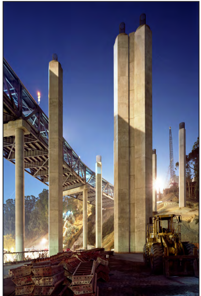
Yerba Buena Island Transition Structures Columns
