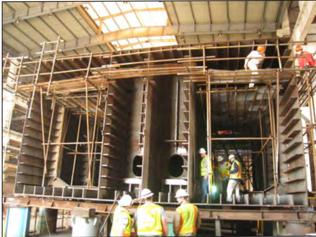
SAS Cross Beam Assembly in Bay 6
