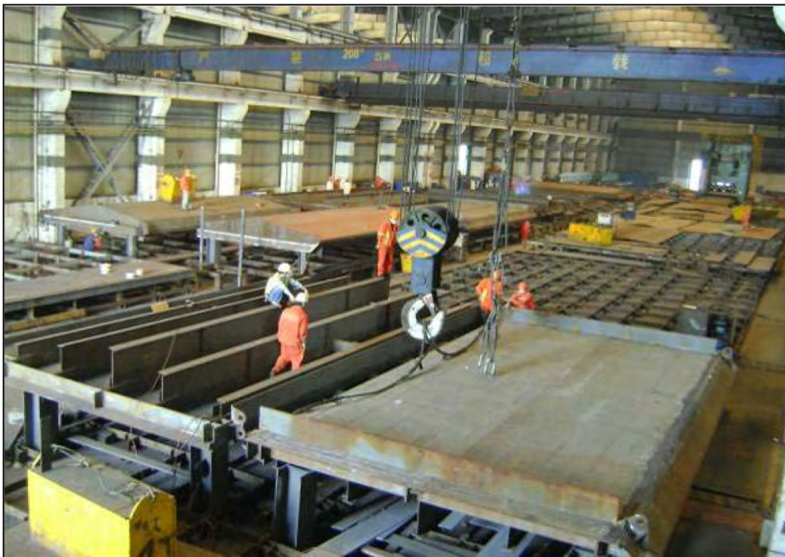
SAS Bike Path Fabrication
