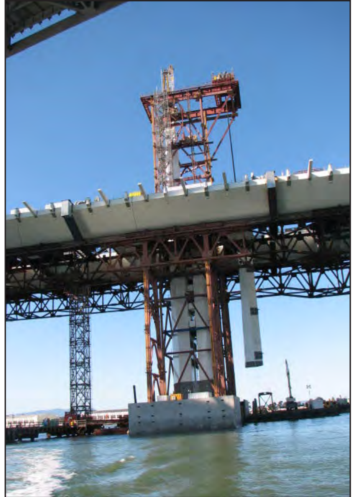
SAS Tower Lift 2 Shafts Being Raised into Position
