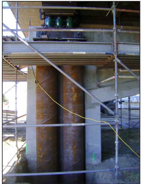
Pier 3 Vertical Lifting Jacks Supported on Temporary Pipe Columns
