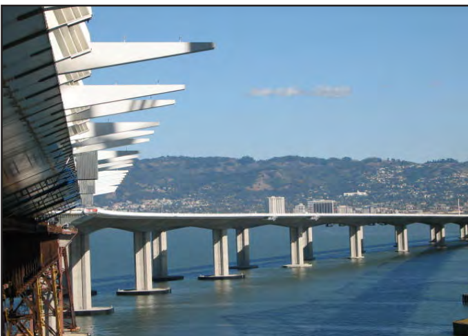
SAS Eastbound Bike Path Support Beams and Skyway
