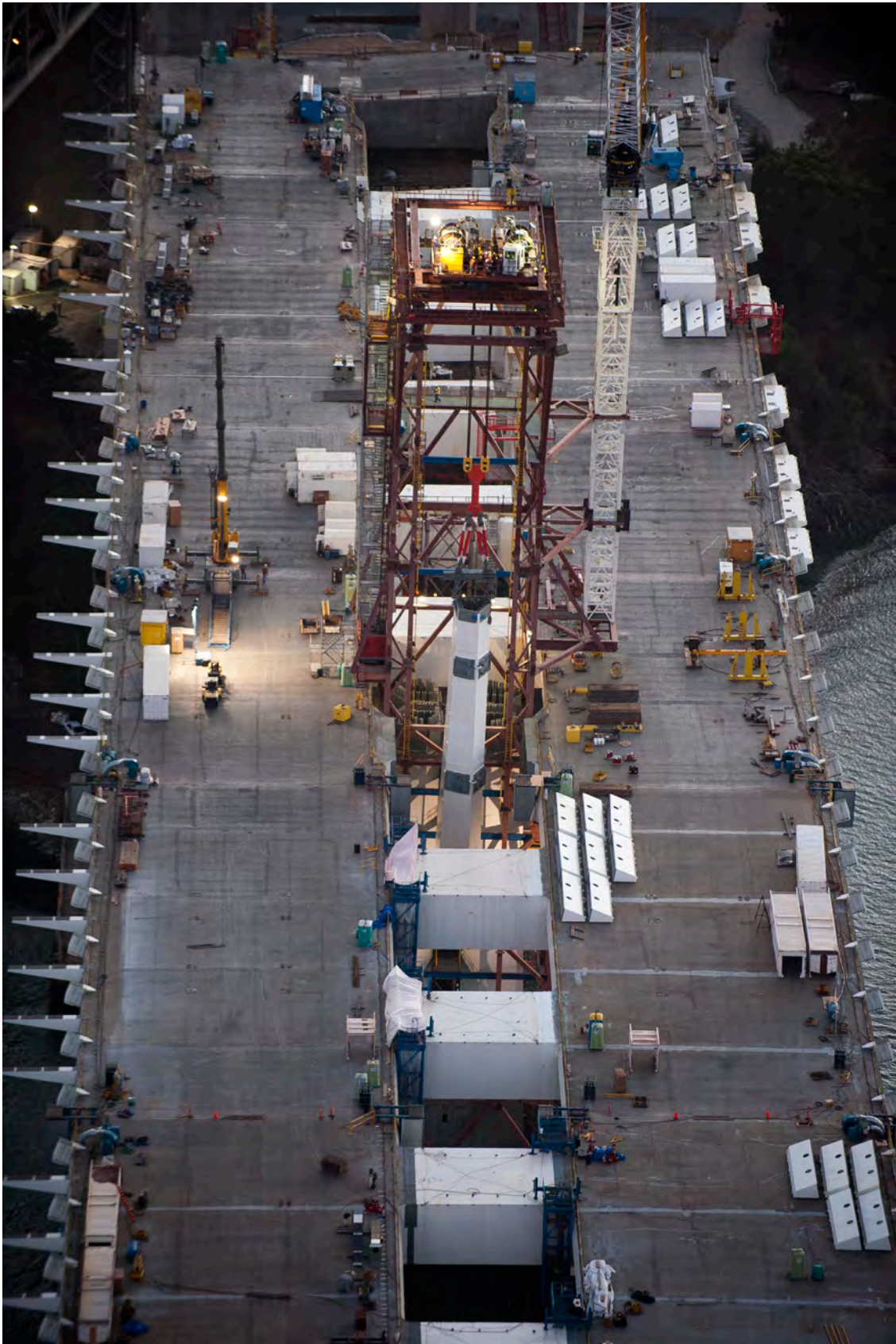
SAS Second Tower Lift
