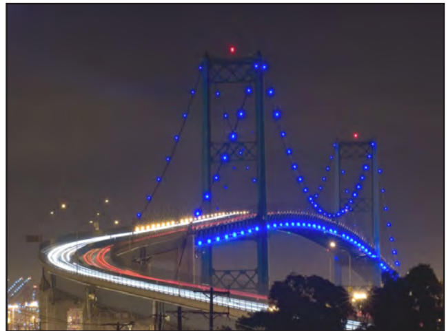
Los Angeles-Vincent Thomas Bridge
