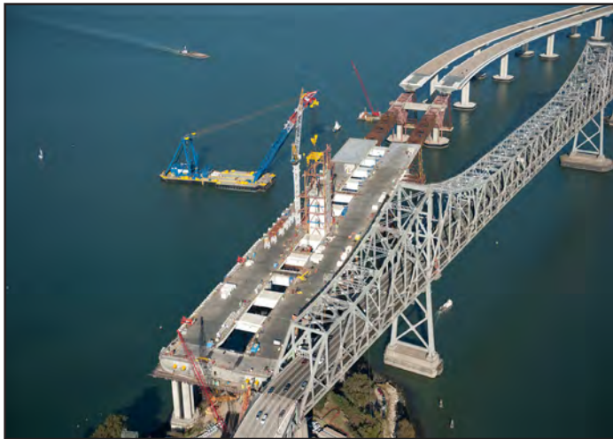
SAS Shear-Leg Crane Barge Lifting Roadway Box 9W
