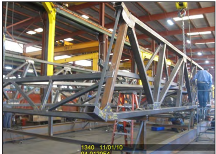
SAS Eastbound Fixed Stair Sections Assembly
