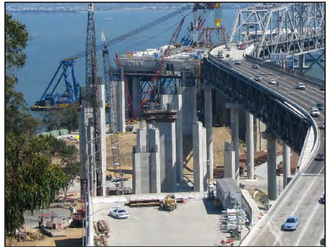
Overview of YBITS Advanced Columns, YBID and SAS W2 Cap Beam
