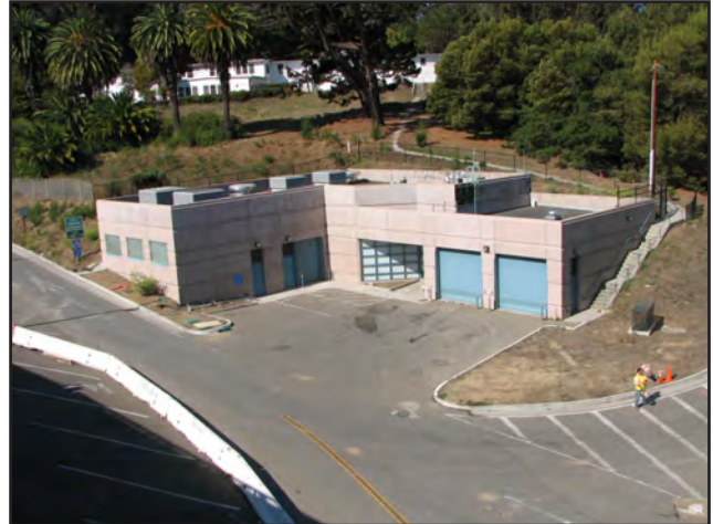
New YBI Electrical Substation
