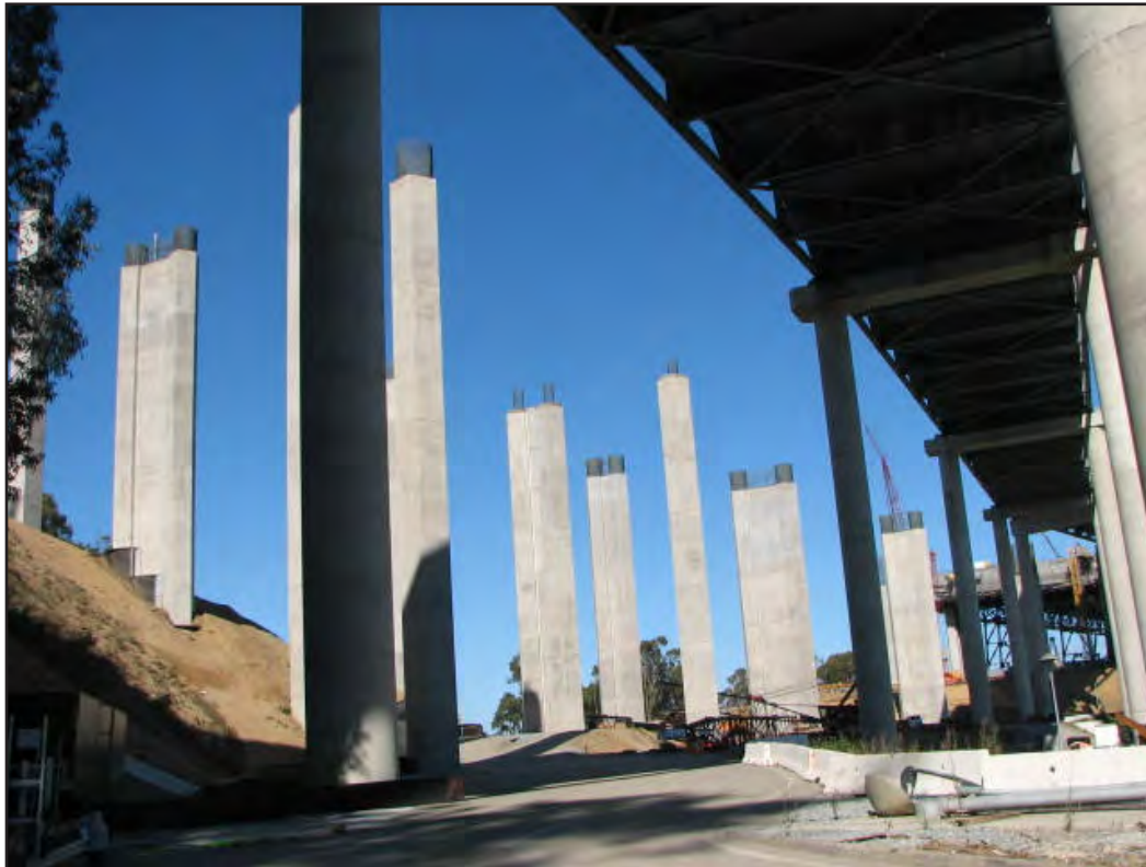
Yerba Buena Island Transition Structures Advanced Columns Constructed
