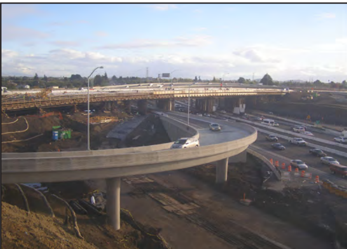
92/880 NWCONN Bridge Construction in Progress
