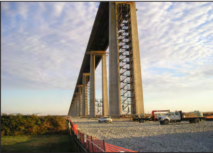
Antioch Bridge Piers Being Fitted for Construction Access Scaffolding
