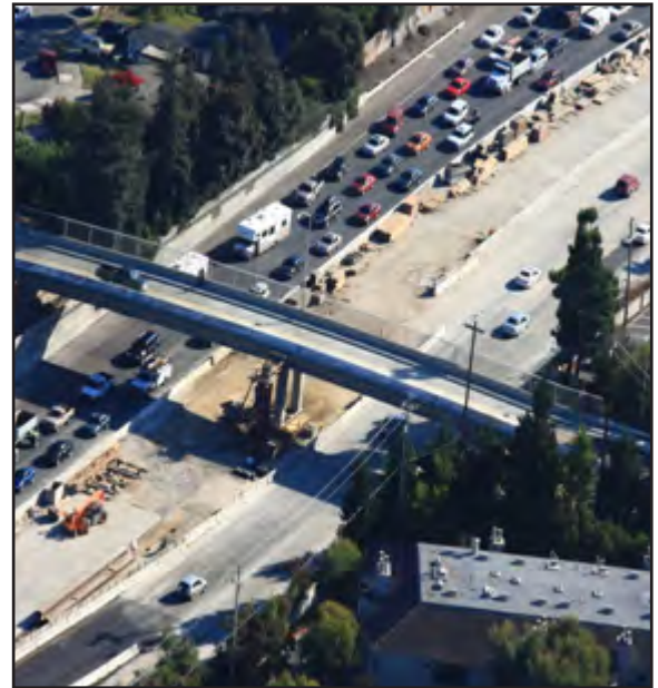
Calaroga Bridge Work in Progress
