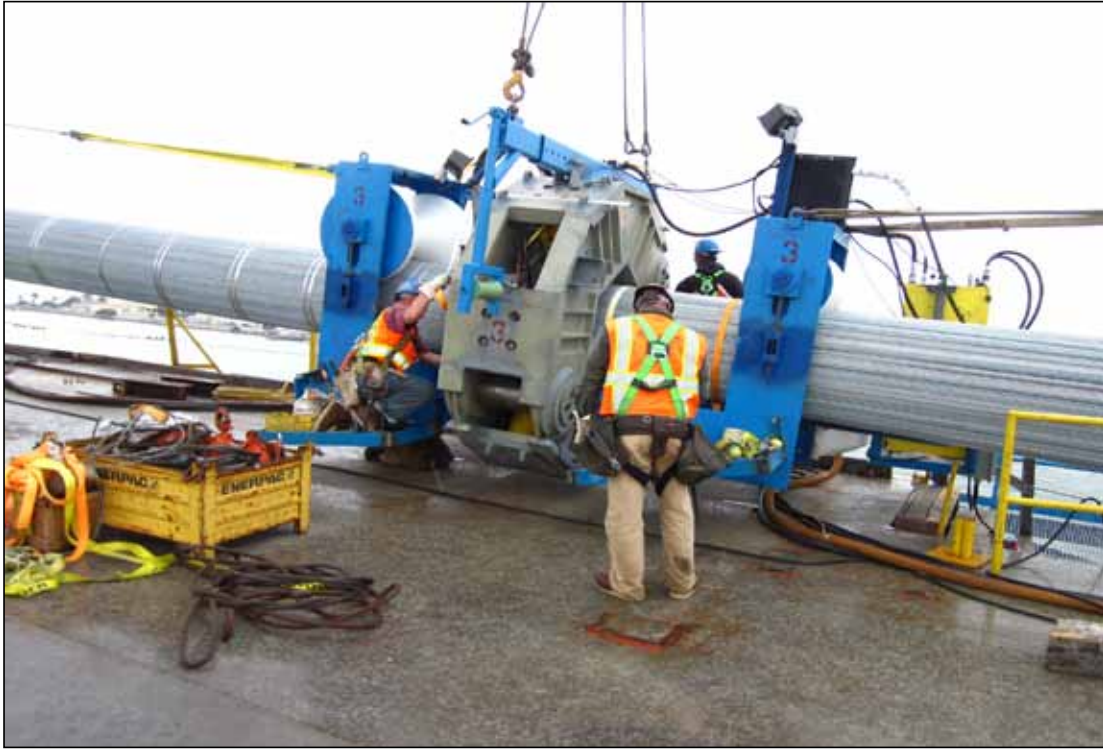
Compacting North Main span PWS Cable Near Completion at East Saddle
