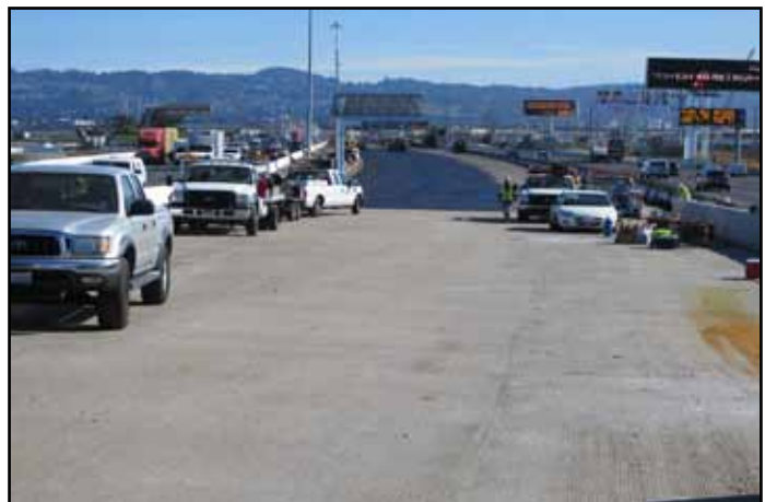
Oakland Westbound Detour (Looking East) AC Asphalt Installed
