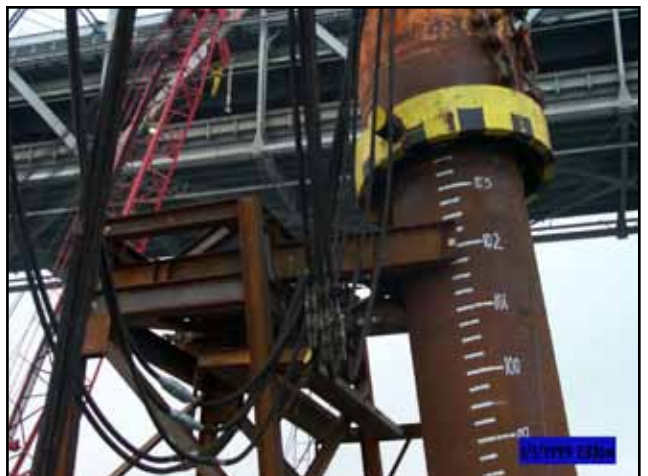
Battered Pile Installation Demonstration
