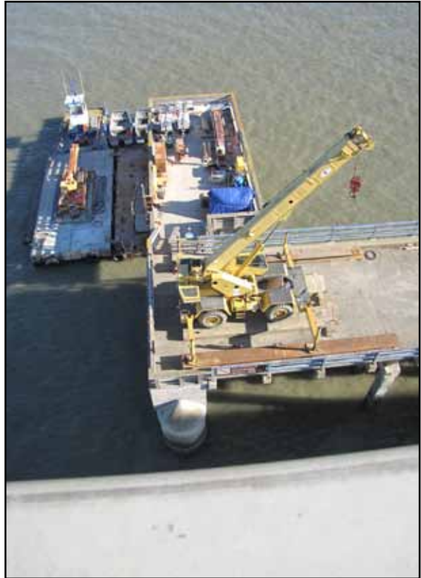
Ravenswood Staging for Footing Overlay Work
