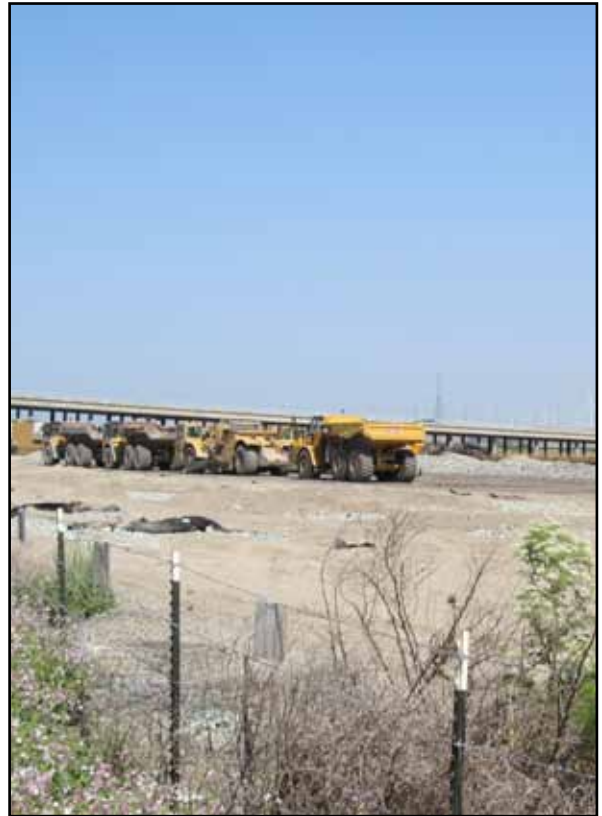
Temporary Contract Yard Removal
