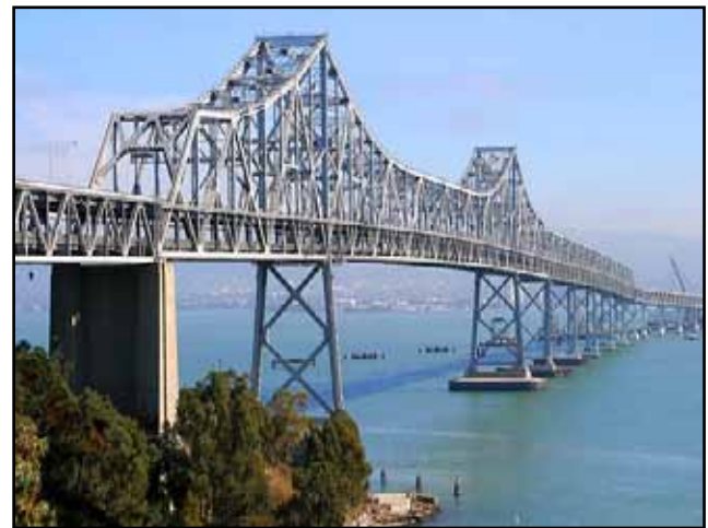
Existing East Span of the San Francisco-Oakland Bay Bridge
