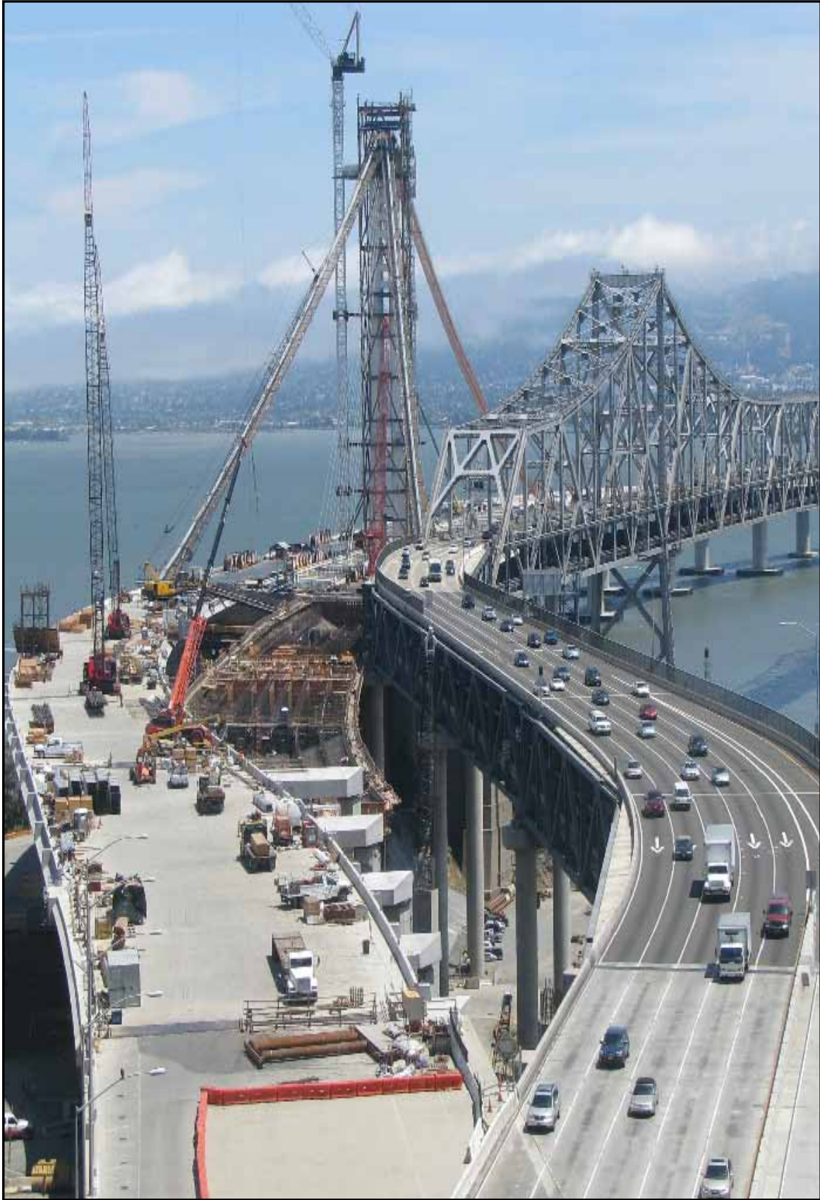
YBITS #1 Westbound Roadway Deck Nearing Completion
