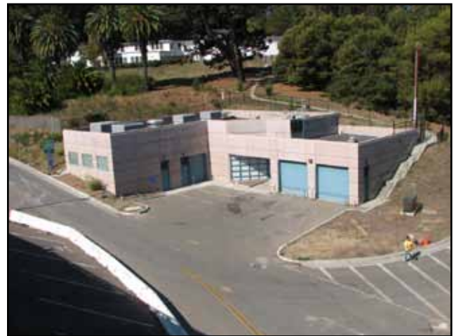
New YBI Electrical Substation
