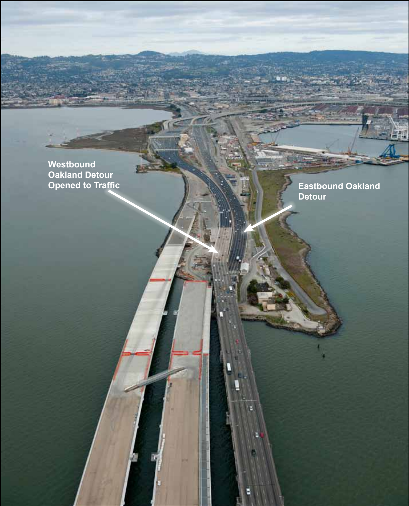
Westbound Oakland Detour Construction Progress
