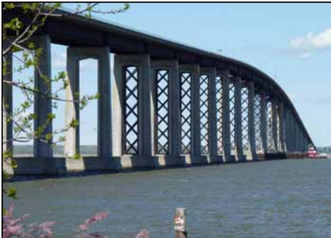
Antioch Bridge Seismic Retrofit
