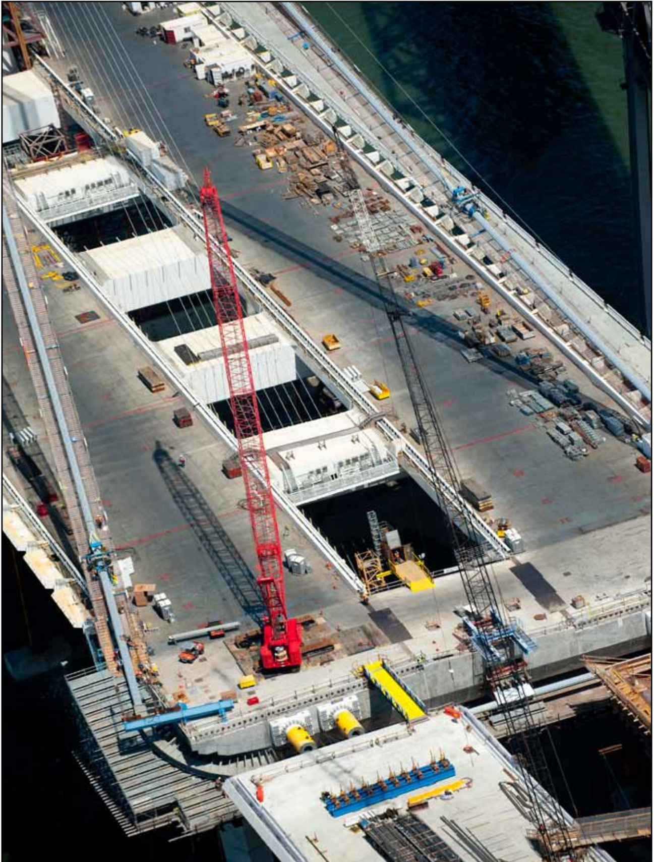
Aerial View Self-Anchored Suspension Bridge and Hinge K Pipe Beams
