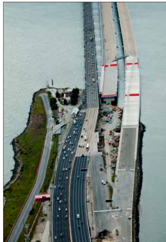
Aerial View of the Eastbound Oakland Detour with the EBMUD Outfall Crossing Structure on the left and the Westbound Oakland Detour Open to Traffic
