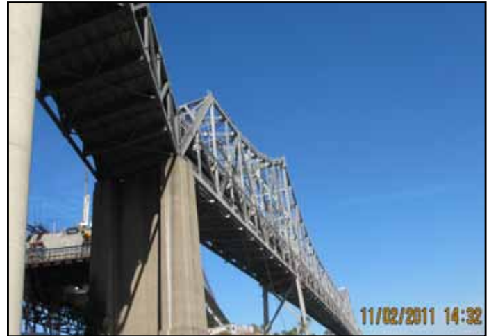
Dismantling Scope Included in the Future YBITS#2 Contract - YBI Detour at left, E-1 column in center, Cantilever Bridge Deck at right
