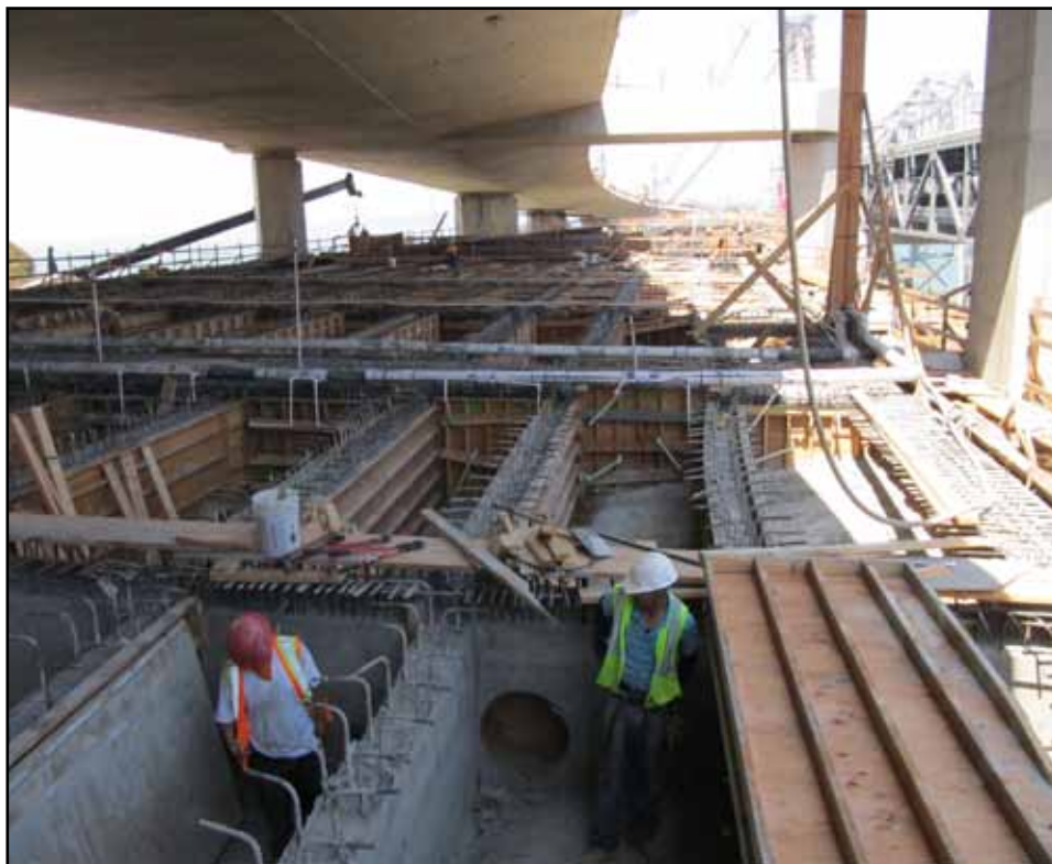
Stripping Stem Wall Forms on YBITS#1 Eastbound
