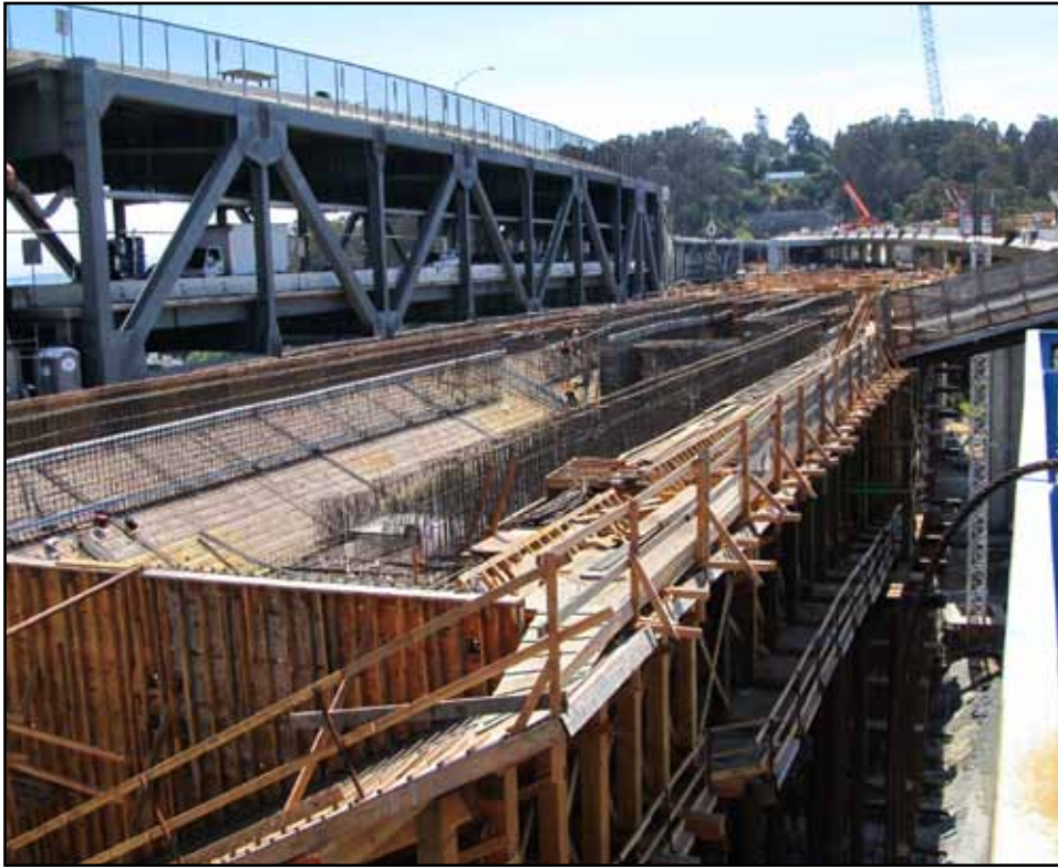
YBITS #1 Soffit Formwork and Rebar Installation in Progress
