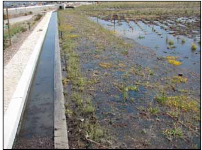
Stormwater Retention Basin
