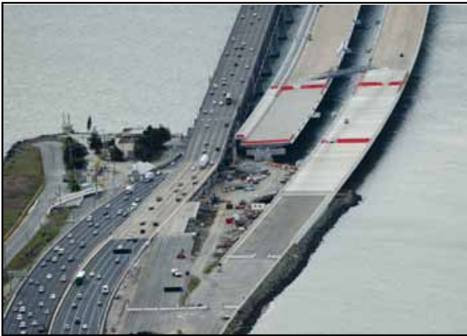
Oakland Detour - Westbound Opened to Traffic
