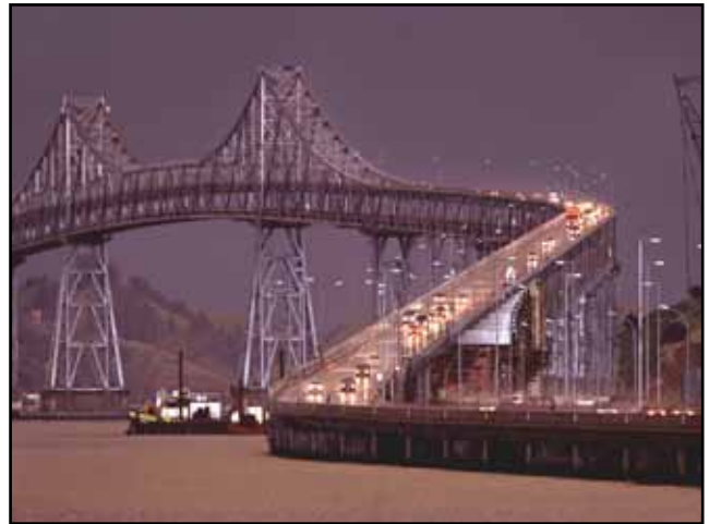
Richmond-San Rafael Bridge
