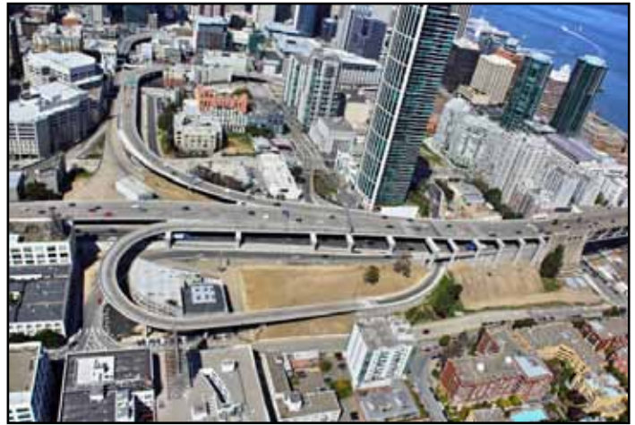
West Approach Overview
