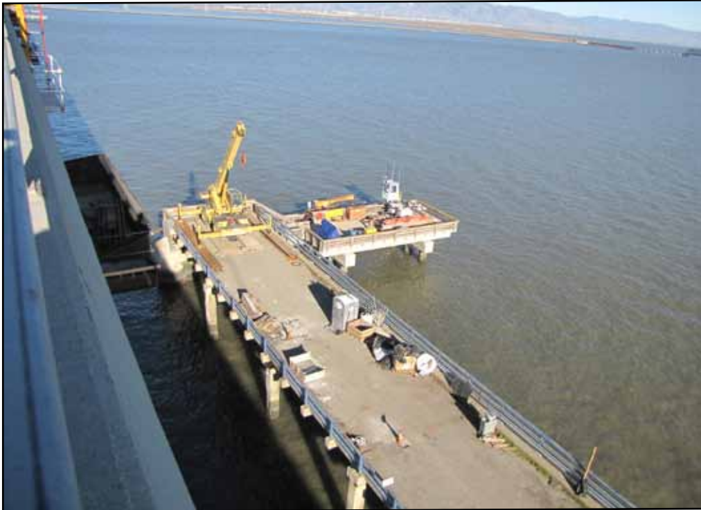
Dumbarton Bridge - Ravenswood Pier Staging for Footing Overlay Work
