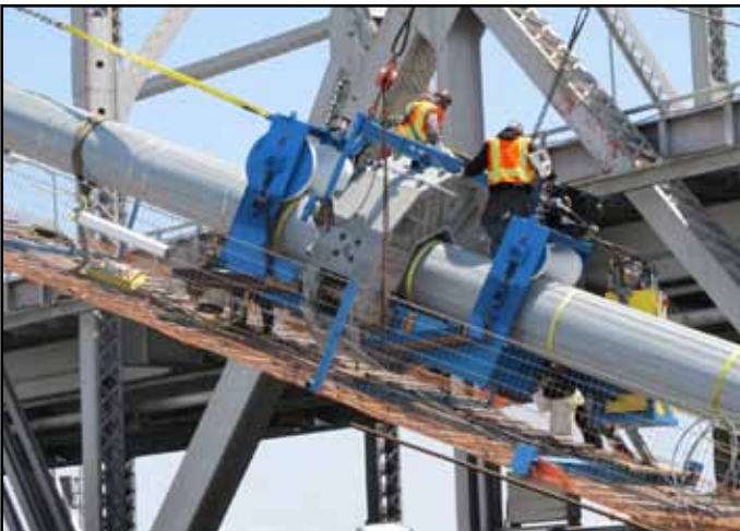
Parallel Wire Strands after Compaction
