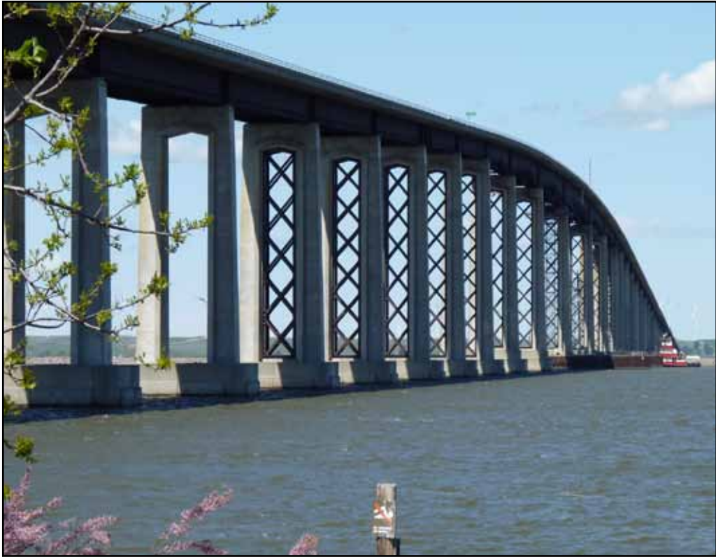
Antioch Bridge with Completed Cross Bracings
