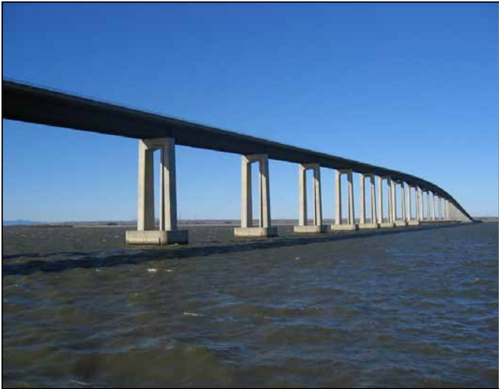
Antioch Bridge Installing Cross Bracing as Part of the Seismic Retrofit Construction
