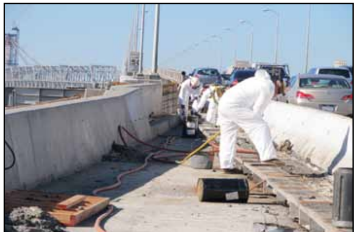
Preparation for Demolition of the Existing Westbound Partial Structure
