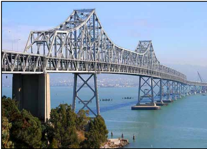
Existing San Francisco-Oakland Bay Bridge Cantilever Section to be Dismantled
