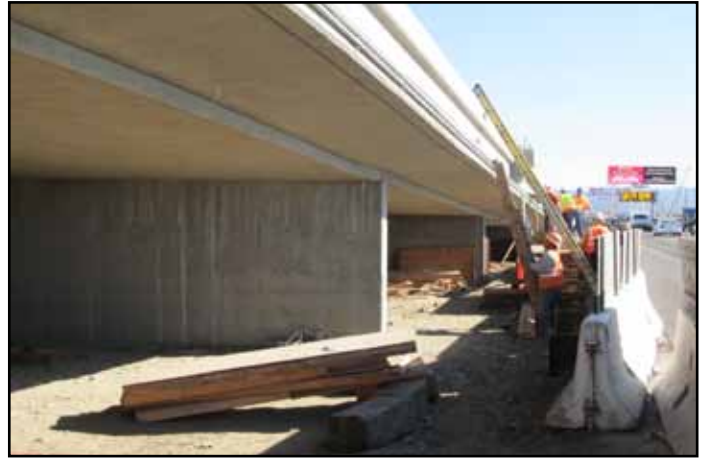
Oakland Detour Westbound Expansion Structure
