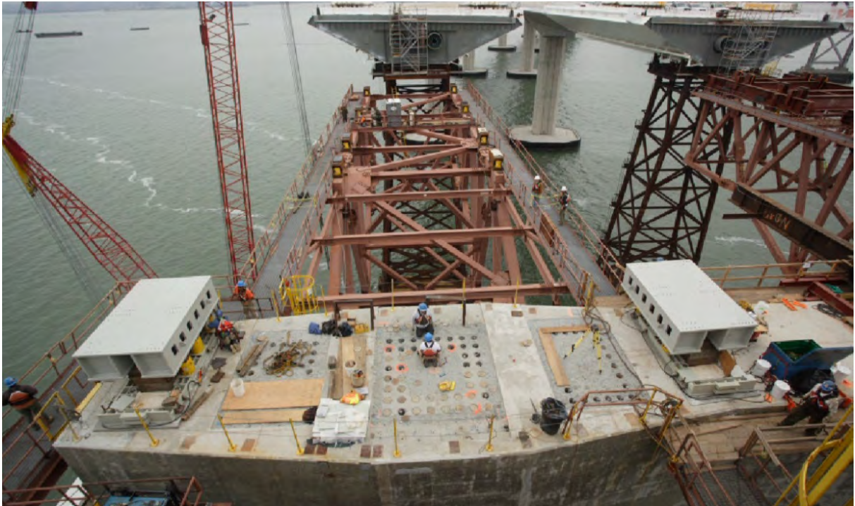
Figure 5 E2 Pier Cap Construction — (Center of photograph is the location of future shear key S1)
