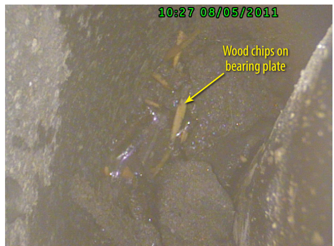
Figure 2.1-10: Various Debris on the Bearing Plate (2)
