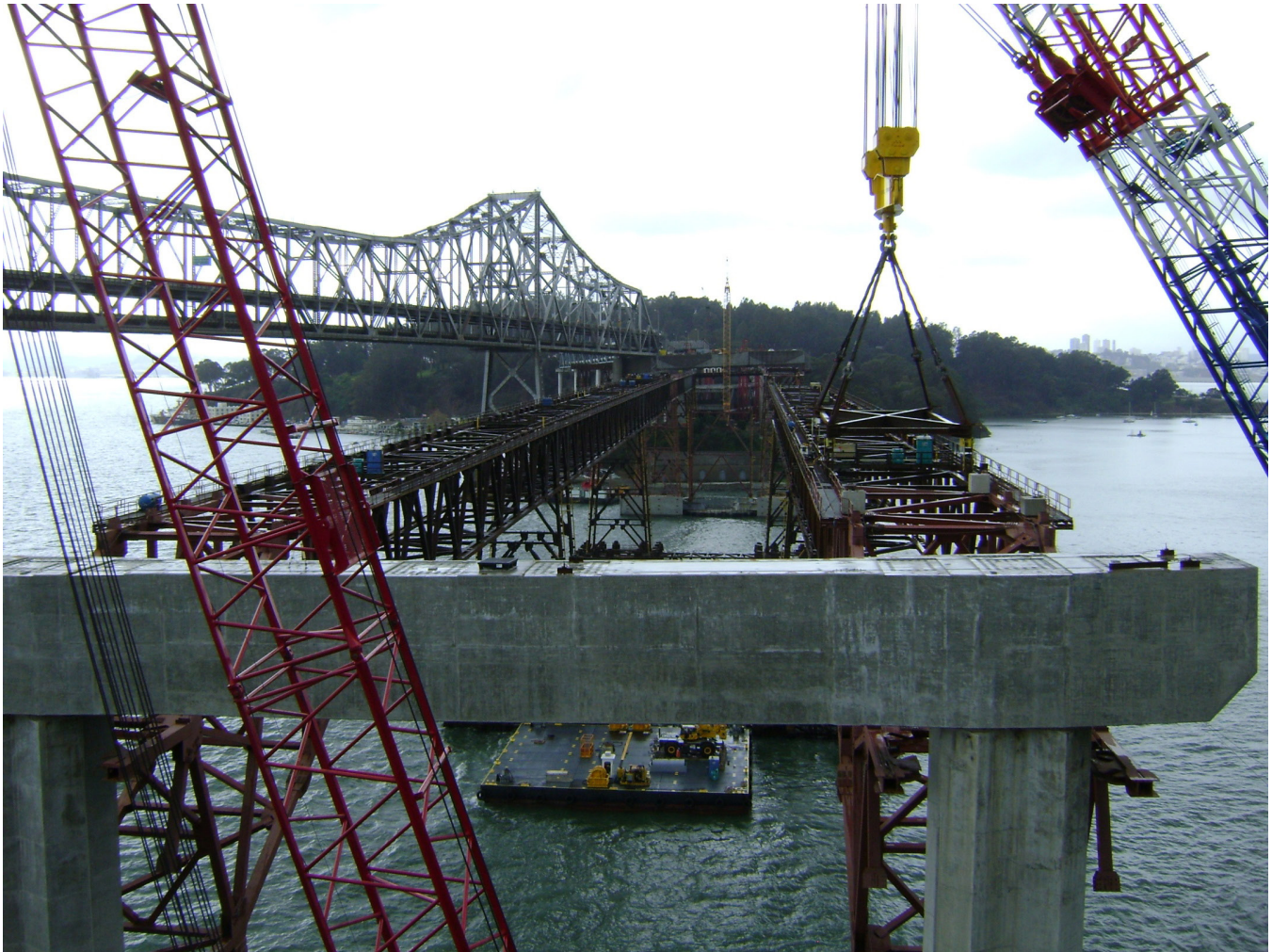
Figure 1.3-1: E2 Cap Beam During Construction (Photo taken 10/19/2009)
