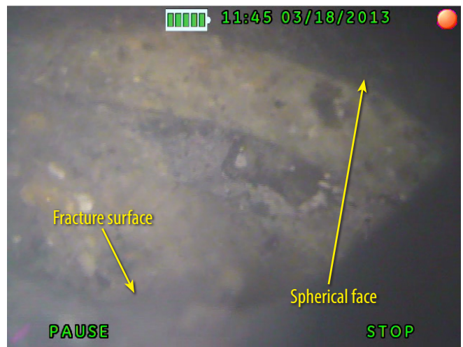
Figure 2.1-17: S2-A8 Borescope Snapshot
