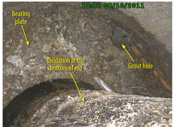
Figure 2.1-10: Various Debris on the Bearing Plate (2)
