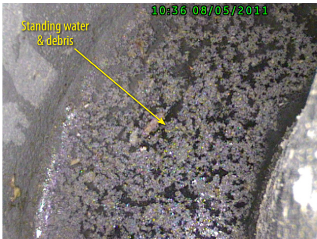
Figure 2.1-9: Various Debris on the Bearing Plate (1)
