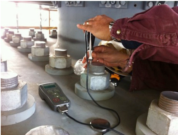
Figure 2.2-1: In-Situ Hardness Testing
