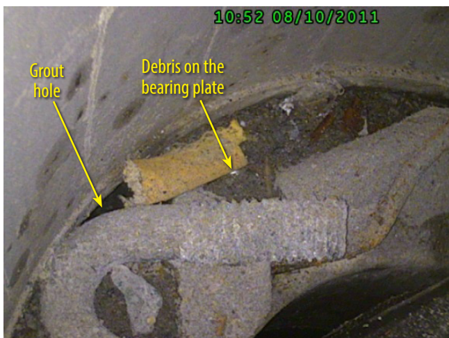
Figure 2.1-9: Various Debris on the Bearing Plate (1)
