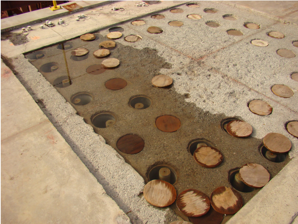
Figure 1.3-3: Shear Keys S1/S2, Rods, Pipe Sleeves, and Top Hat Details
