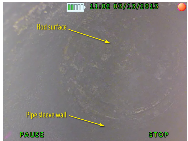
Figure 2.1-13: S2-A6 Borescope Snapshot
