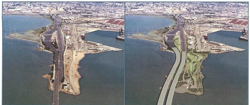
The proposed Gateway Park will transform the current barren land at the Oakland Touchdown Area into a park allowing for spectacular views of the Bay. The picture on the right is one concept EBRPD is proposing for the new park.
