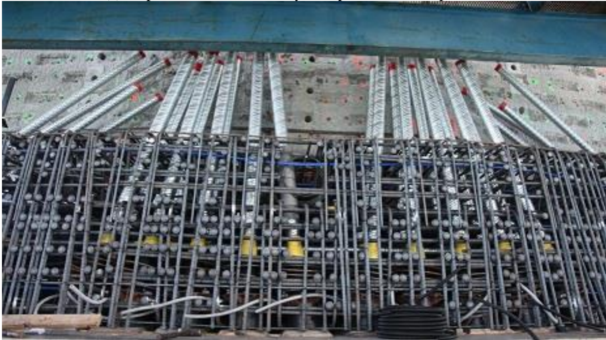
(b) Rebars and PT tendons for holding the saddles down to the E2 cap beam
