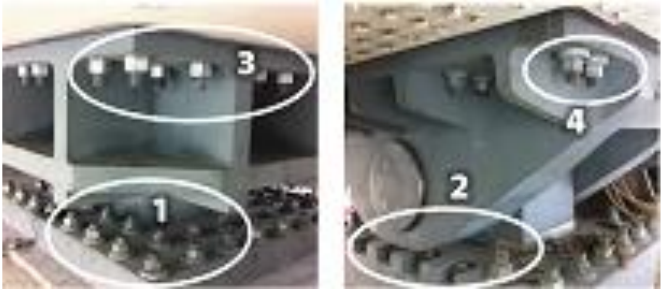
(a) 1 – Shear key, base plate anchor rods 3 – Shear key, top rods
