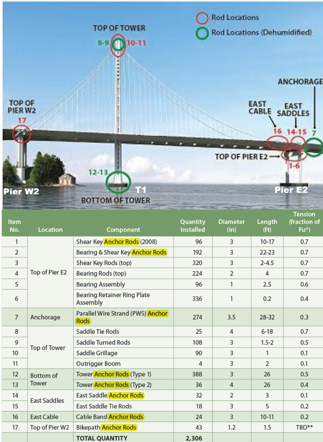
Figure 2 Identification of ASTM A354 Grade BD rods on the SAS Bridge.
