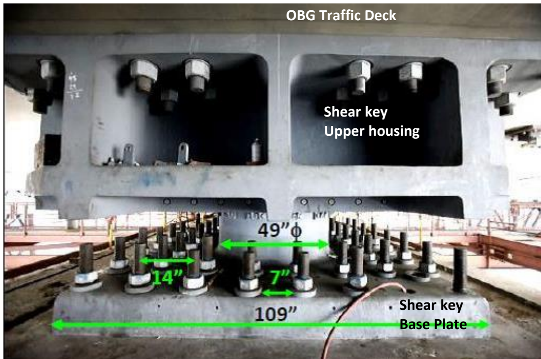
(a) Anchor rod lay out for shear key base plate
