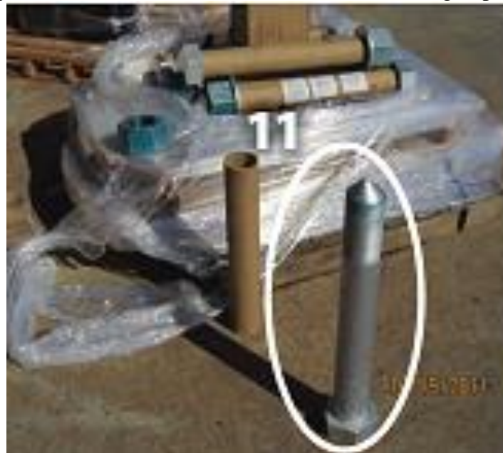
(c) 11 – Outrigger boom anchor rod at tower top 107
