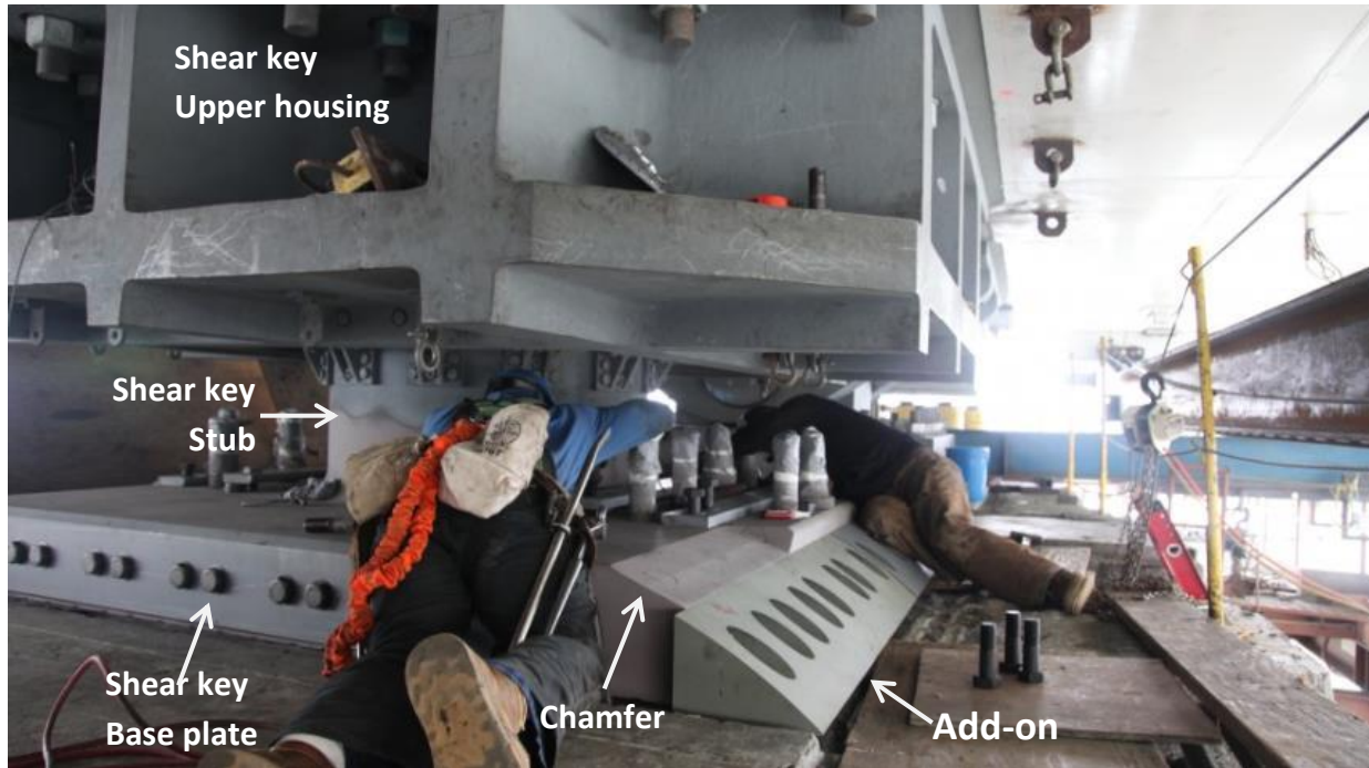
(a) Preparation of the shear key base plate for saddle placement
